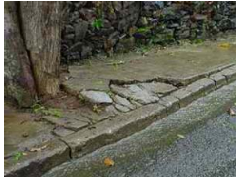
P-4 Deformation on the sidewalk
