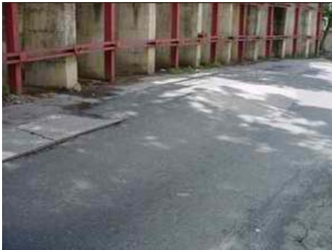
P-3 Deformation on the road
