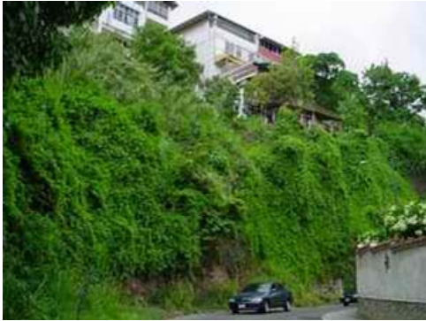
P-1 View of North part of the slope
