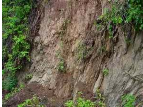
P-4 Surface collapse
