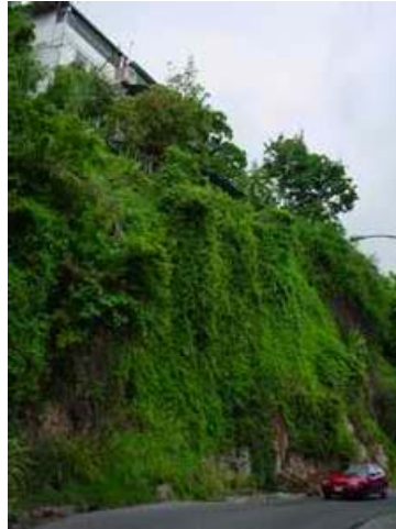
P-2 View of South part of the slope
