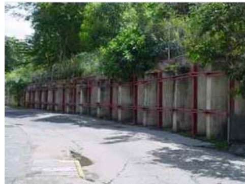
P-4 Cracks on the road
