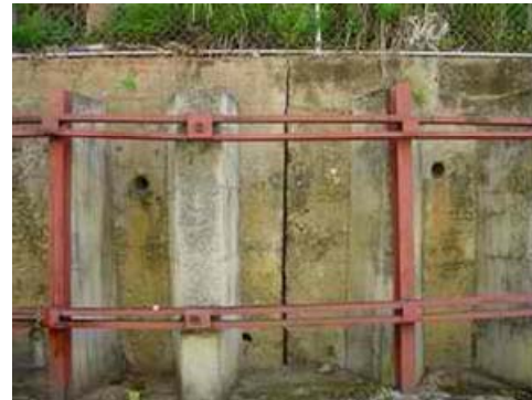
P-6 Crack on the concrete wall
