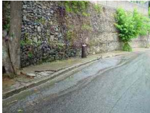
P-2 Deformation on the road
