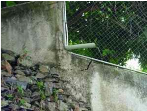
P-3 Crack on the concrete wall
