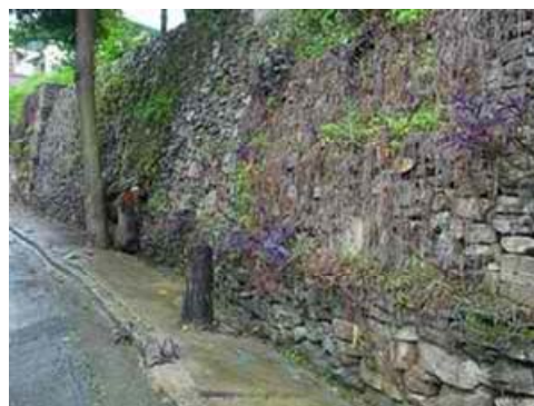
P-5 Bulging at toe of the block wall
