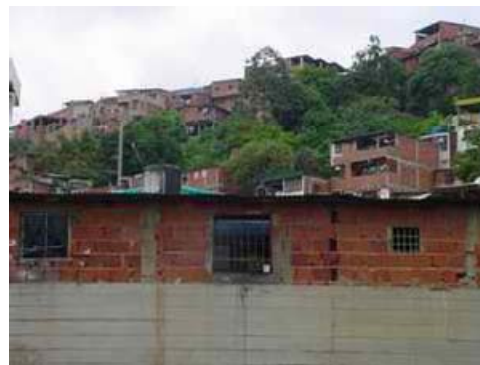
P-4 View of South part of the slope
