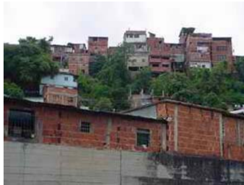
P-2 View of North part of the slope
