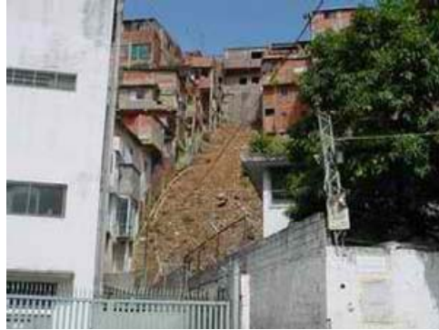
P-2 The bare slope situation
