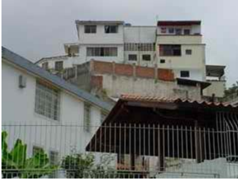
P-1 View of West part of the slope
