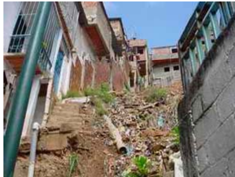
P-4 Close view for the bare slope
