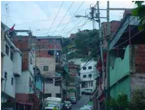
P-1 View of South part of the slope
