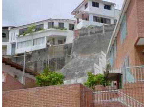
P-2 Existing Countermeasure (Concrete Wall)
