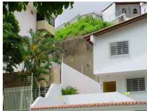
P-4 Existing Countermeasure (Concrete Wall+Anchor work)
