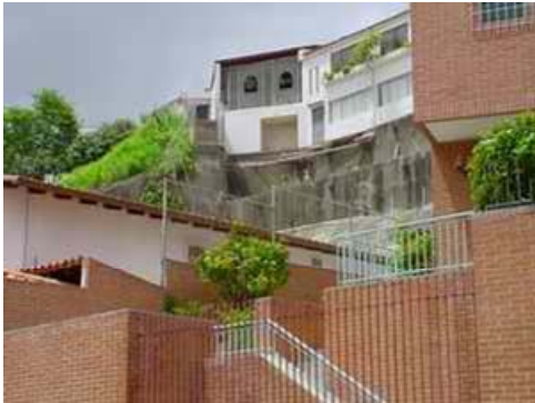
P-3 Existing Countermeasure (Concrete Wall)
