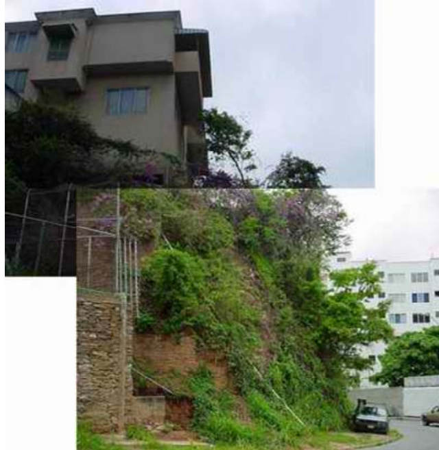
P-1 Situation of the cut slope (South part of the slope)
