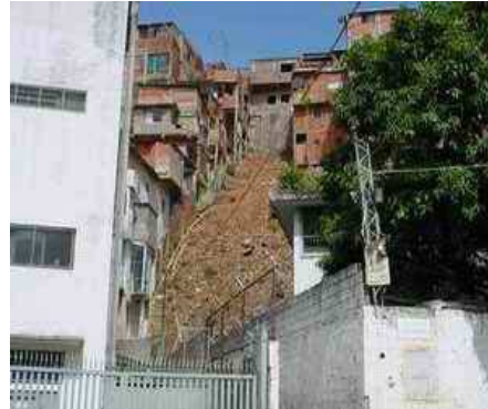
P-2 The bare slope situation
