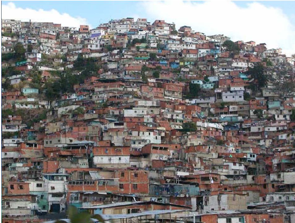
Figure S21-1.2.1 Caracas Hillside Barrio
