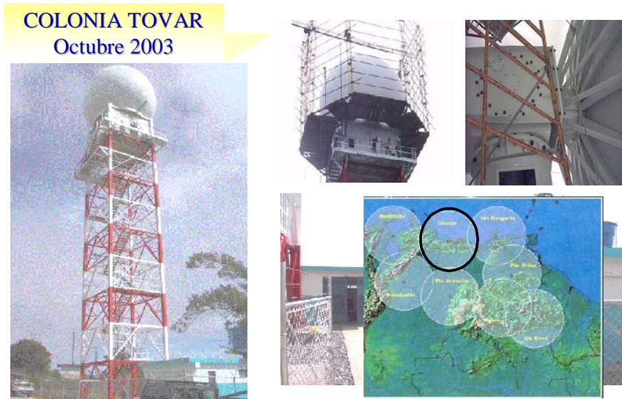
Figure S18-2.3.2 Meteorology Radar Installed in Colonia Tovar to Cover the Entire Caracas Valley (Source: MARN)
