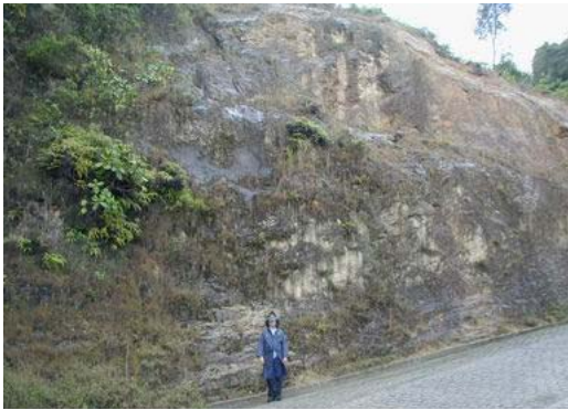
Weathering Grade V – IV Upper one third of this slope is Grade V
