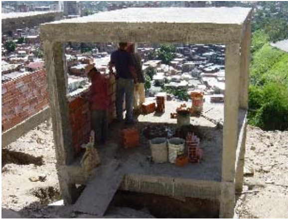
Photo 3.37 Clay Brick Wall Work (1)
