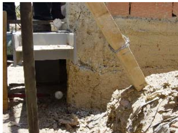
Photo 6.12 Model 3-Diagonal Shear Crack of Short Column
