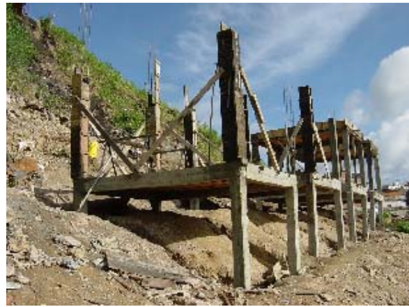
Photo 3.34 Column Form Work (2)
