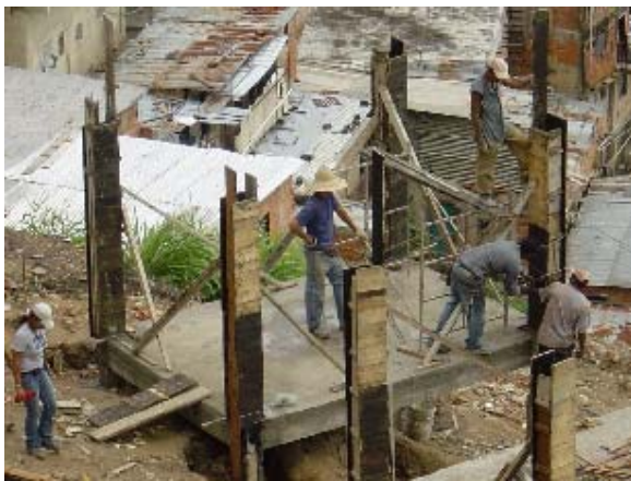
Photo 3.33 Column Form Work (1)
