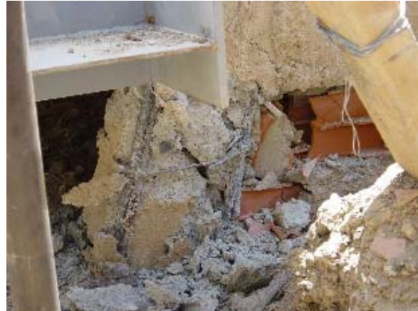
Photo 6.13 Shear Failure of Column and Clay Brick Wall (1)
