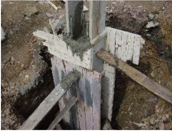
Photo 3.19 Short Column Form Work(1)
