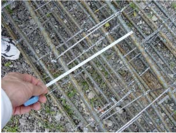
Photo 3.13 Fabrication of Re-bars(1)
