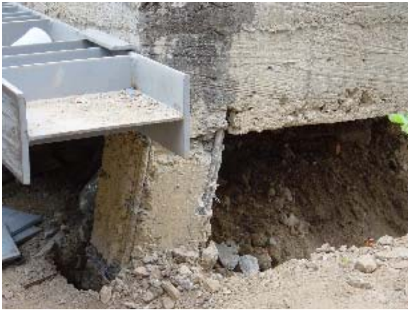
Photo 6.1 Model 1-Short Column Failure (1)
