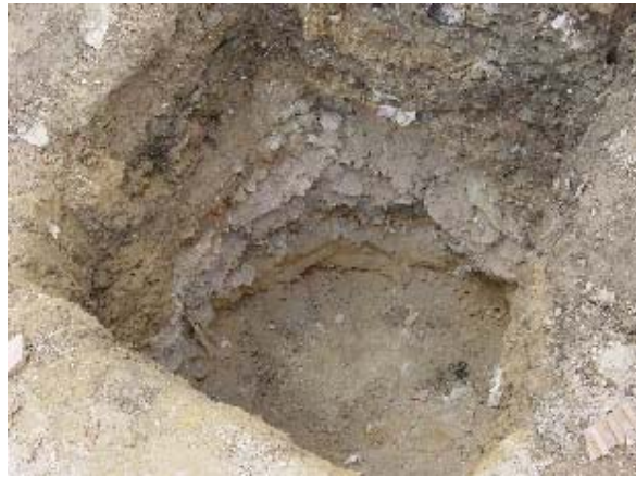
Photo 3.16 Excavation for Foundation
