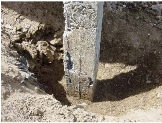
Photo 6.9 Model 2-Long Column Failure
