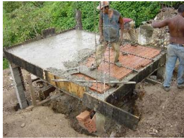
Photo 3.32 Tabela Floor and Concreting
