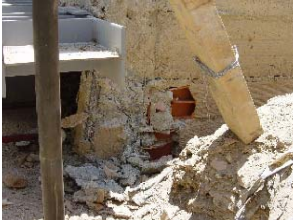
Photo 6.13 Shear Failure of Column and Clay Brick Wall (1)
