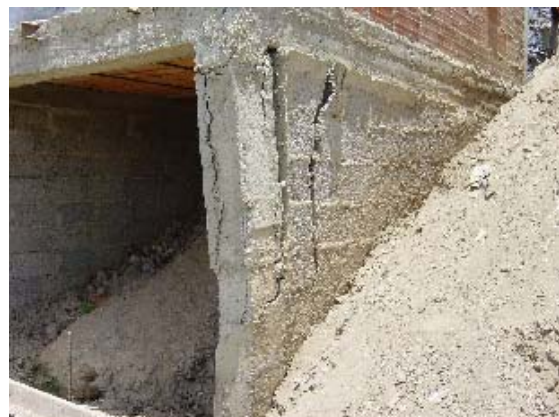
Photo 6.17 Separation of Concrete Block Wall without Re-bars from Frame
