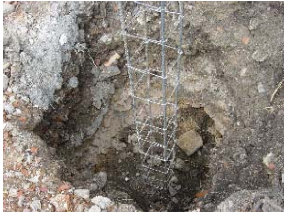
Photo 3.18 Short Column Re-bar
