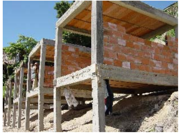
Photo 3.38 Clay Brick Wall Work(2)
