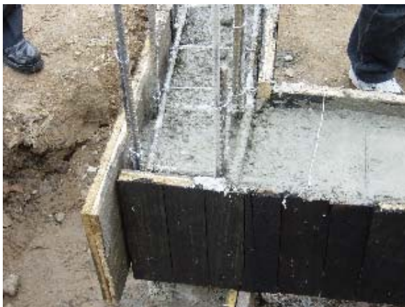
Photo 3.29 Construction Joint at beam
