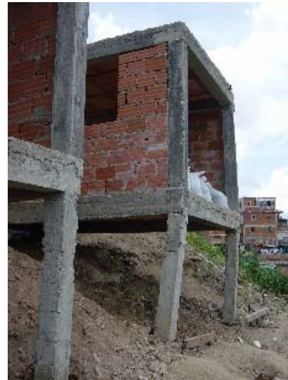
Photo 6.4 Model 1-Long Column Failure
