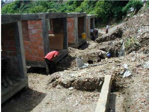
Photo 3.43 Retaining Wall
