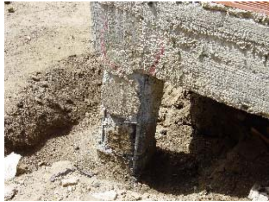
Photo 6.8 Model 2-Shear Crack of Short Column (3)
