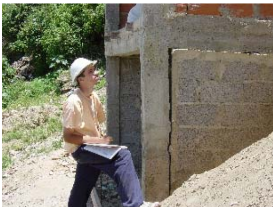
Photo 6.17 Separation of Concrete Block Wall without Re-bars from Frame
