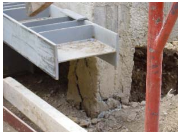
Photo 6.6 Model 2-Shear Failure of Short Column (1)
