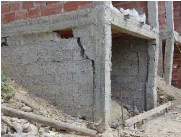
Photo 6.21 Failure of Concrete Block Wall with Re-bars
