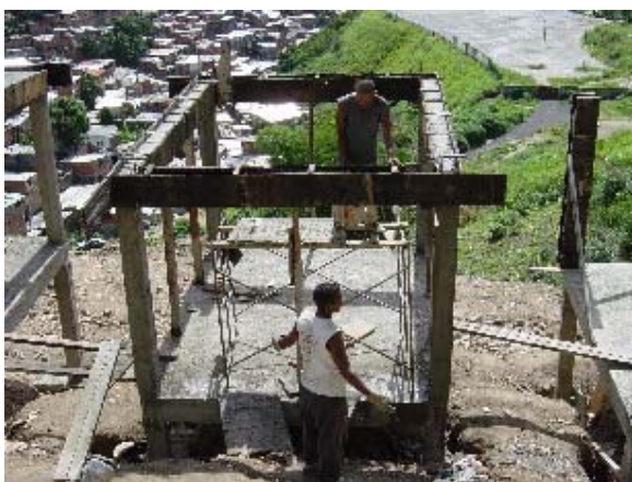
Photo 3.35 Roof Beam Form Work
