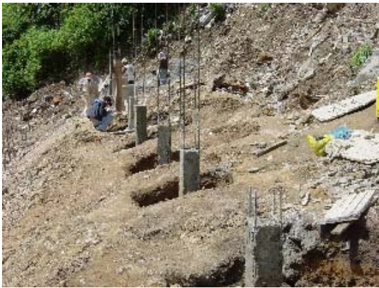
Photo 3.23 Short Column Concreted(2)
