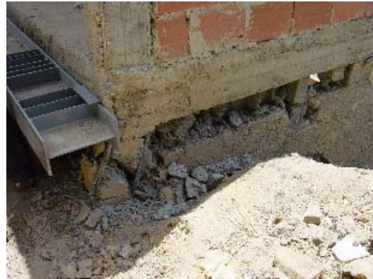
Photo 6.19 Shear Failure of Column and Concrete Block wall with Re-bars (1)
