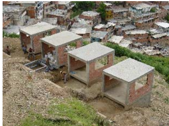
Photo 3.8 Brick Wall work
