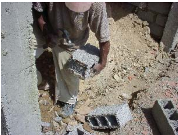
Photo 3.41 Concrete Block Wall Work(1)
