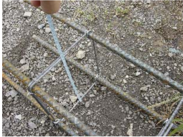
Photo 3.14 Fabrication of Re-bars(2)
