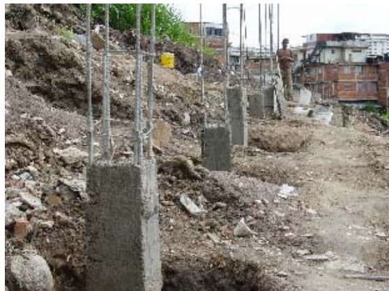
Photo 3.24 Short Column Concreted(3)
