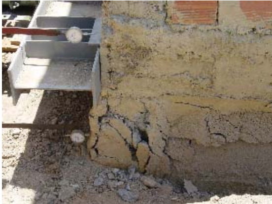
Photo 6.19 Shear Failure of Column and Concrete Block wall with Re-bars (1)
