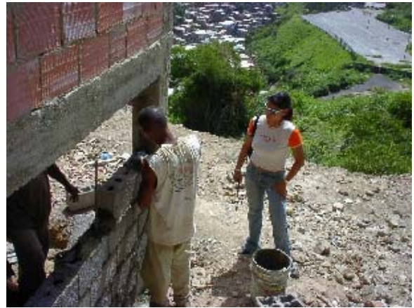
Photo 3.42 Concrete Block Wall Work(2)
