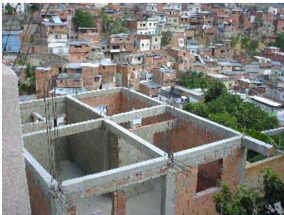
Photo 1.3 A Barrio house under construction
