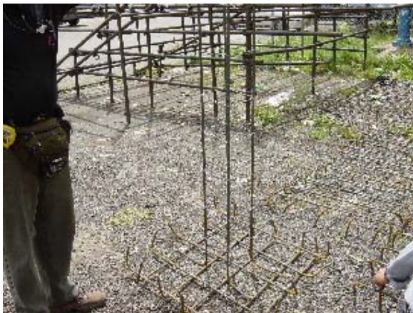
Photo 3.15 Fabrication of Re-bars(3)
