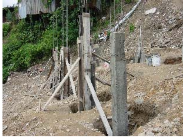
Photo 3.26 Long Column Concreted
