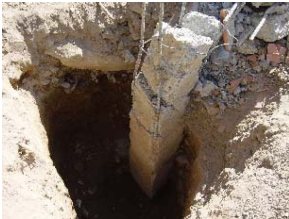
Photo 6.3 Model 1-Short Column Failure (3)
