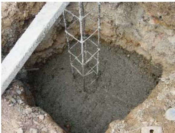
Photo 3.17 Concrete Casting for Foundation
