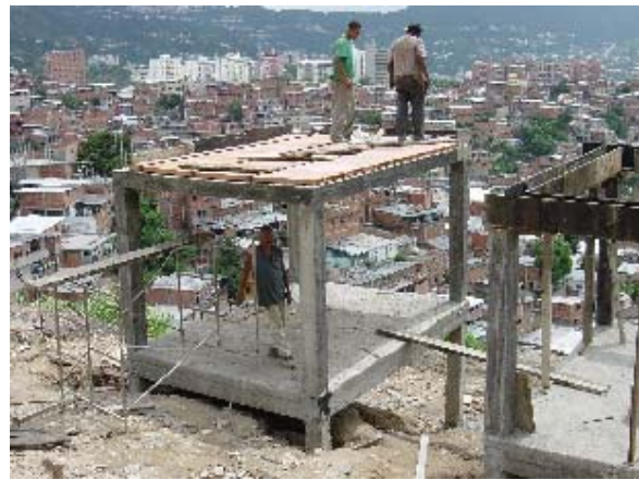
Photo 3.36 Roof Floor Work
