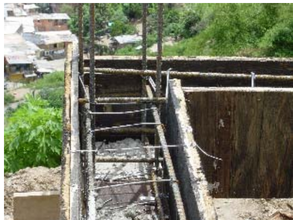
Photo 3.28 Beam Re-bar Installation
