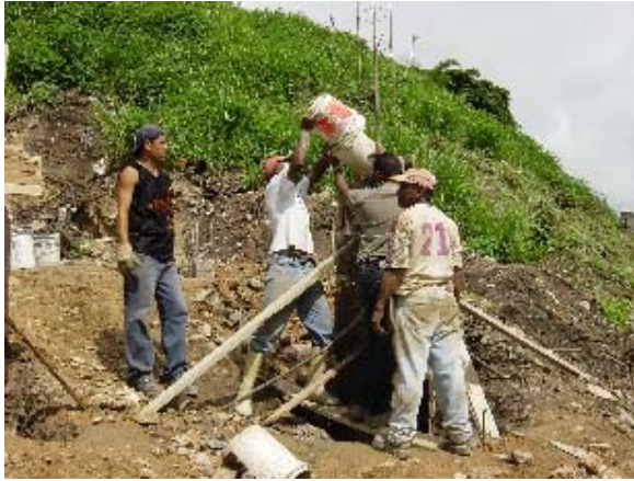
Photo 3.25 Long Column Concreting
