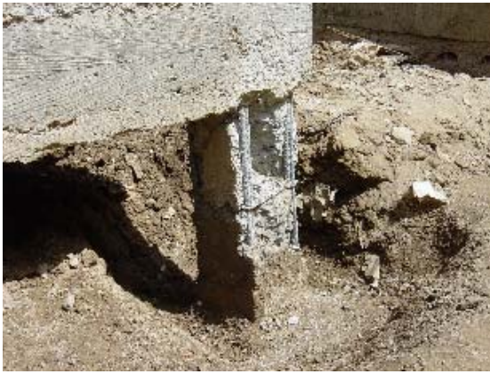
Photo 6.7 Model 2-Shear Failure of Short Column (2)
