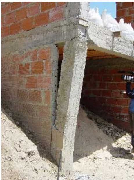
Photo 6.15 Separation of Wall and Frame
