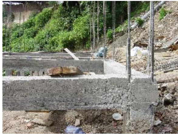
Photo 3.30 Removal of Form Work
