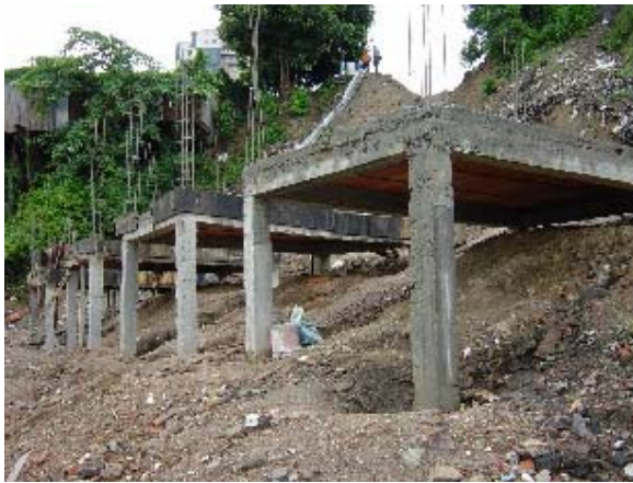
Photo 3.31 Long Column and Floor
