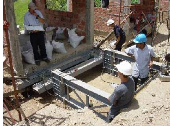
Photo 5.2 Steel Frame for Load Transfer
