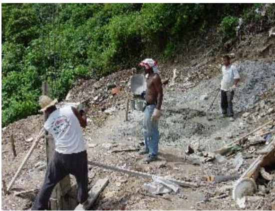
Photo 3.21 Short Column Concreting
