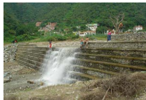
Existing Sabo Dam in San Jose de Galipan
