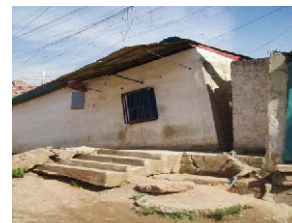
Damaged House in Antimano
