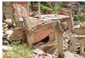
Damaged House in 19 de Abril
