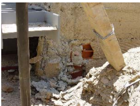
Photo 3.5.68 Shear Failure of Column and Clay Brick Wall (1)
