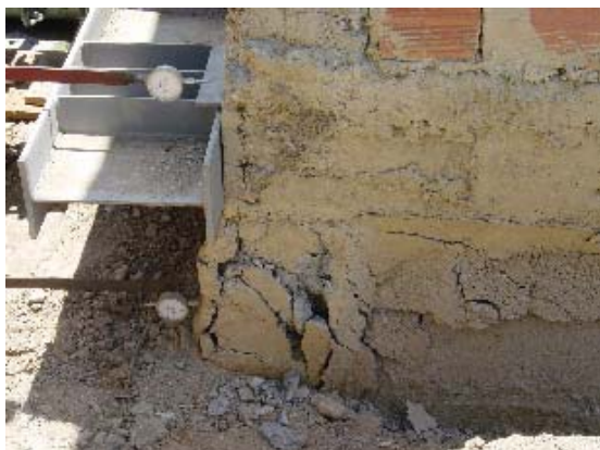
Photo 3.5.74 Shear Failure of Column and Concrete Block wall with Re-bars(1)
