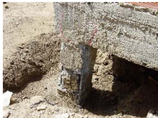
Photo 3.5.62 Model 2-Shear Failure of Short Column (2) Photo 3.5.63 Model 2-Shear Crack of Long Column
