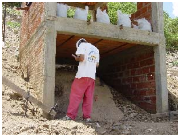
Photo 3.5.66 Model 3 Photo 3.5.67 Model 3-Diagonal Shear Crack of Short Column
