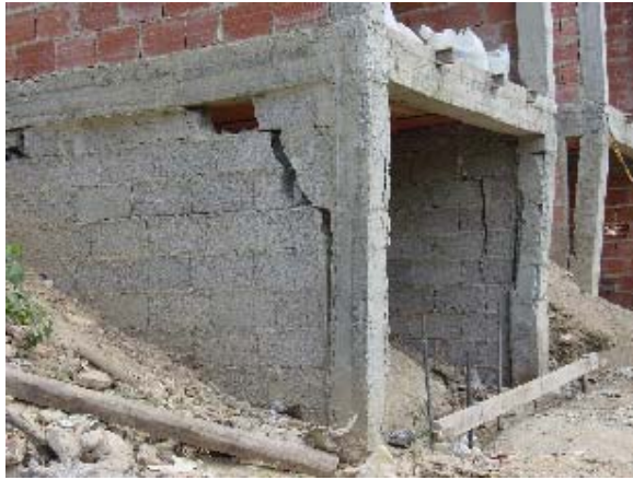
Photo 3.5.76 Failure of Concrete Block Wall with Re-bars
