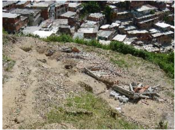
Photo 3.5.76 Failure of Concrete Block Wall with Re-bars
