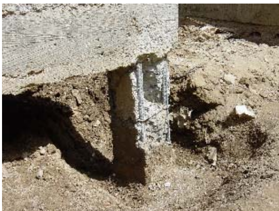
Photo 3.5.62 Model 2-Shear Failure of Short Column (2) Photo 3.5.63 Model 2-Shear Crack of Long Column
