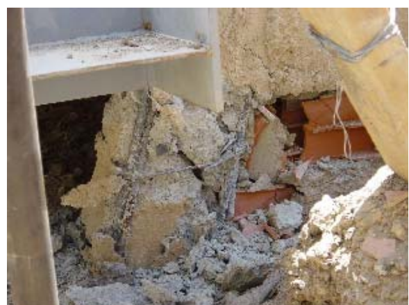
Photo 3.5.68 Shear Failure of Column and Clay Brick Wall (1)
