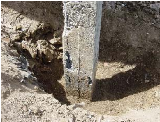
Photo 3.5.64 Model 2-Long Column Failure (2)
