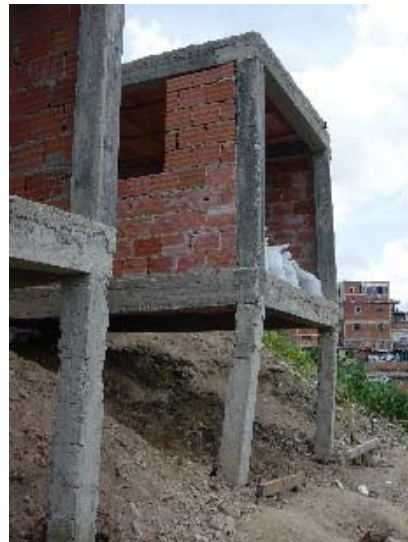
Photo3.5.58 Model 1 Short Column Failure(3) Photo3.5.59 Model1 Long Column Failure
