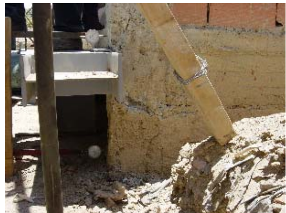
Photo 3.5.65 Model 2-Short Column under Grade Beam
