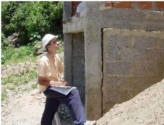
Photo 3.5.72 Separation of Concrete Block Wall without Re-bars from Frame
