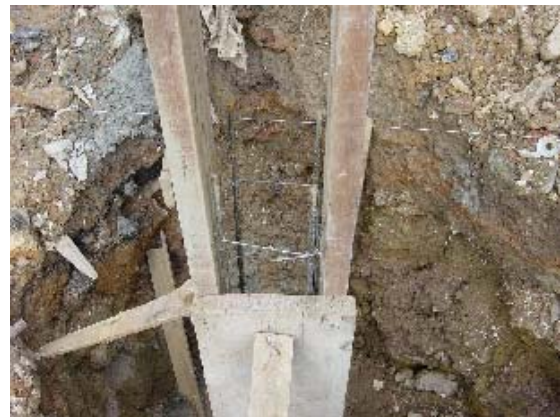
Photo 3.5.24 Short Column Form Work(1) Photo 3.5.25 Short Column Form Work(2)
