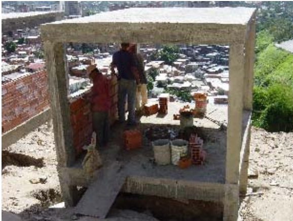
Photo 3.5.42 Clay Brick Wall Work (1)
