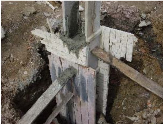
Photo 3.5.24 Short Column Form Work(1) Photo 3.5.25 Short Column Form Work(2)
