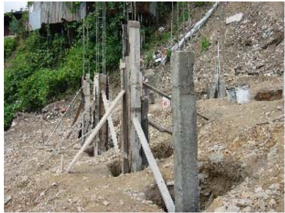
Photo 3.5.31 Long Column Concreted
