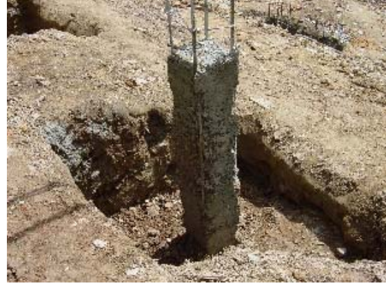
Photo 3.5.24 Short Column Form Work(1) Photo 3.5.25 Short Column Form Work(2)
