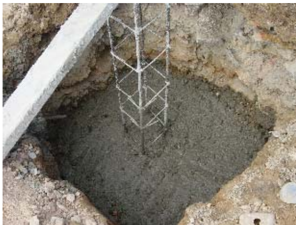
Photo 3.5.22 Concrete Casting for Foundation
