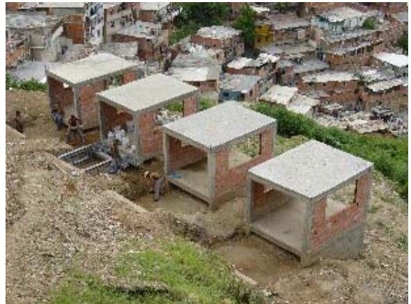
Photo 3.5.13 Brick Wall work
