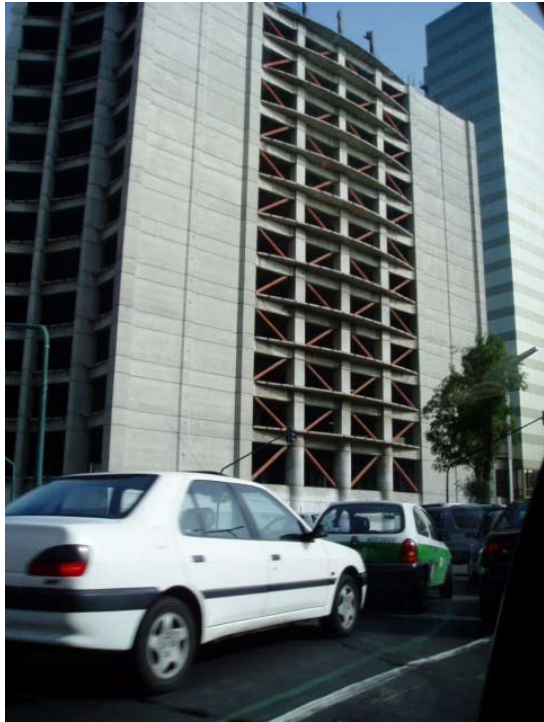
Figure 3.5.24 Sample of Steel Bracing Reinforcement
