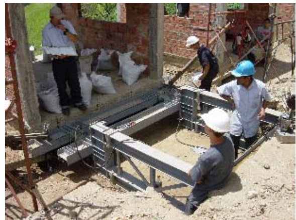
Photo 3.5.51 Steel Frame for Load Transfer
