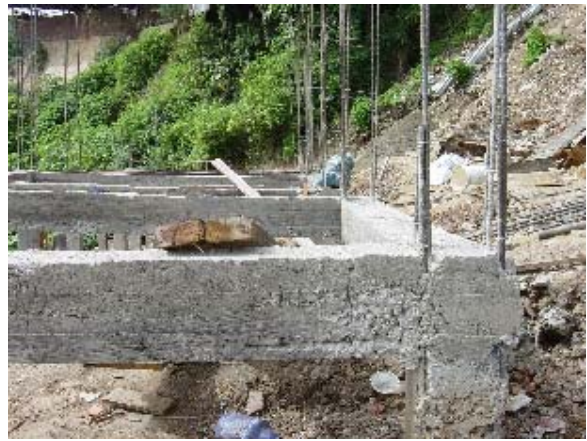
Photo 3.5.35 Removal of Form Work
