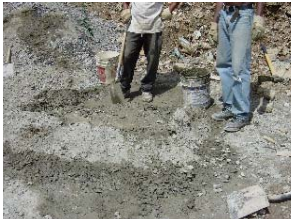
Photo 3.5.14 Concrete Mixing
