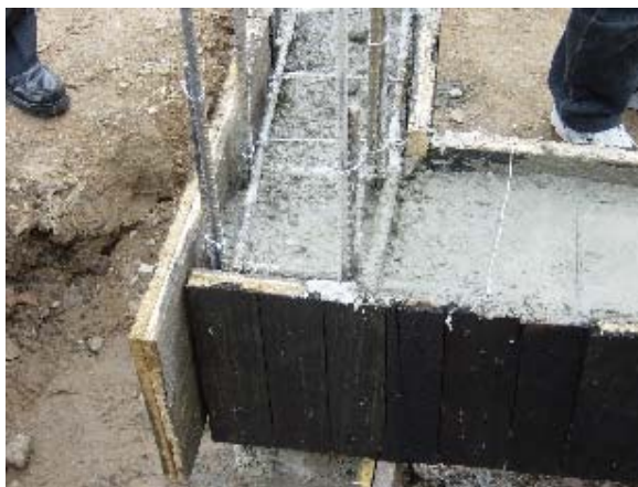
Photo 3.5.34 Construction Joint at beam
