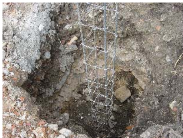
Photo 3.5.23 Short Column Re-bar
