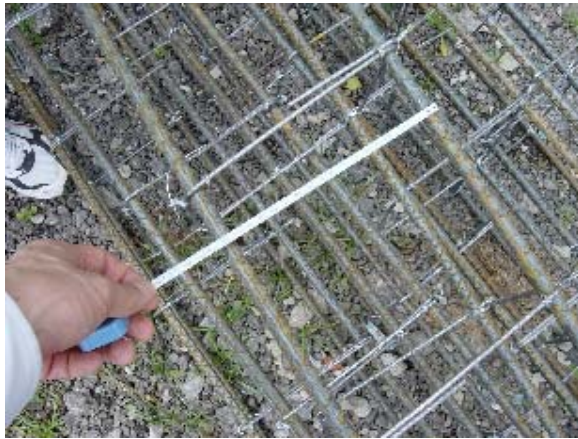
Photo 3.5.18 Fabrication of Re-bars(1)
