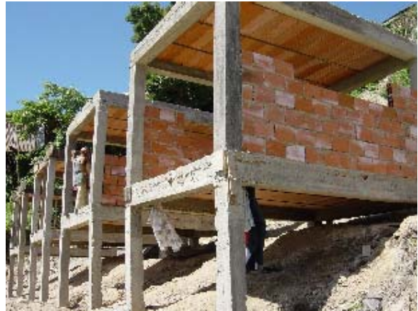
Photo 3.5.43 Clay Brick Wall Work(2)
