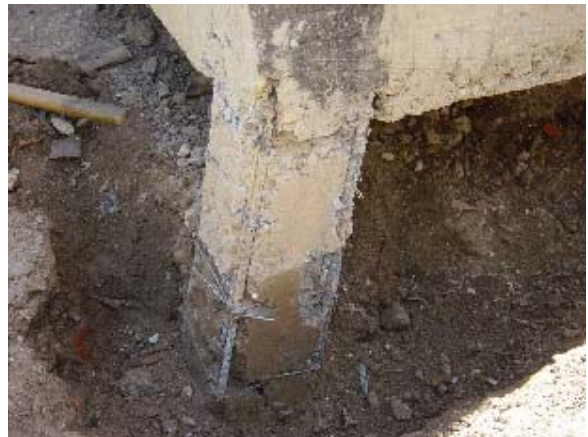
Photo3.5.57 Model 1-Short Column Failure(2)
