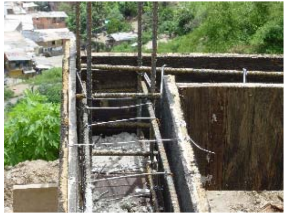
Photo 3.5.33 Beam Re-bar Installation
