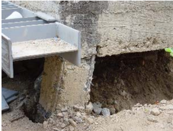
Photo 3.5.56 Model 1-Short Column Failure (1)
