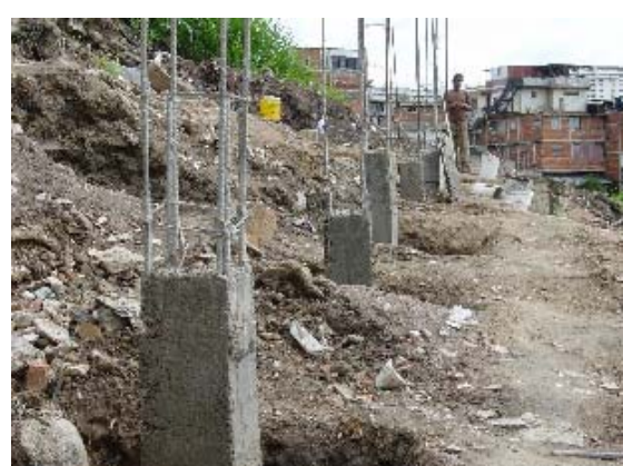
Photo 3.5.26 Short Column Concreting Photo 3.5.27 Short Column Concreted(1)
