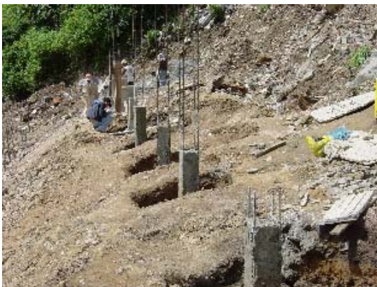
Photo 3.5.26 Short Column Concreting Photo 3.5.27 Short Column Concreted(1)
