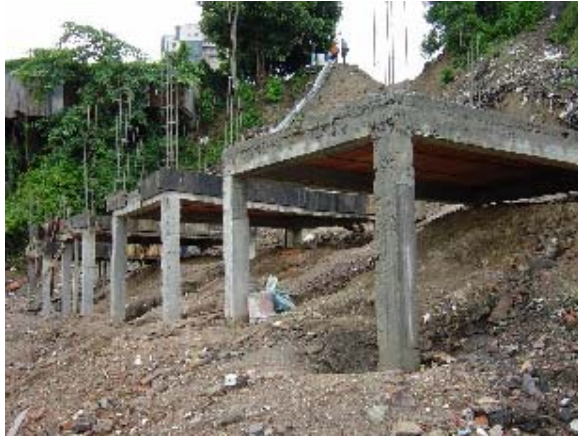
Photo 3.5.36 Long Column and Floor
