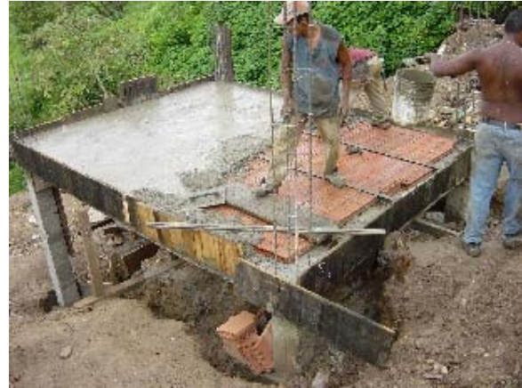
Photo 3.5.37 Tabelone Floor and Concreting
