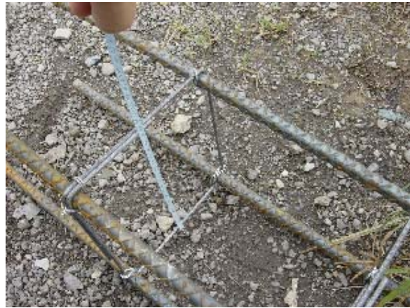
Photo 3.5.19 Fabrication of Re-bars(2)
