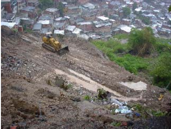
Photo 3.5.6 Site Grading Work
