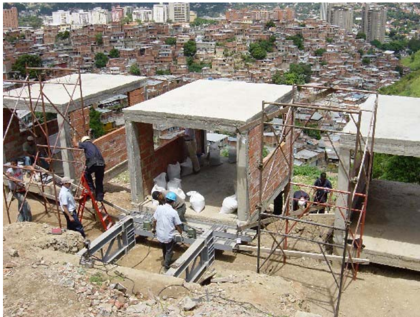
Photo 3.5.3 Horizontal Loading by Hydraulic Jack
