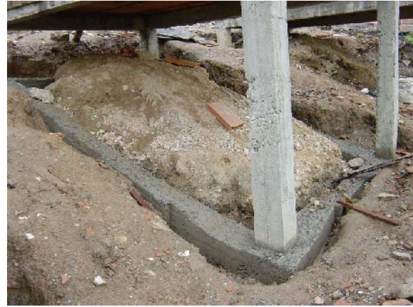
Photo 3.5.2 Grade Beams
