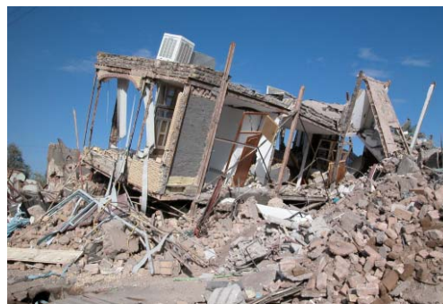
Figure 2.2.3 Example of a Totally Collapsed Building of Steel Frame
