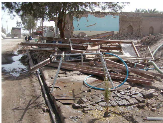
Photo 2.3.1 Tap Water connected to Main Pipe
