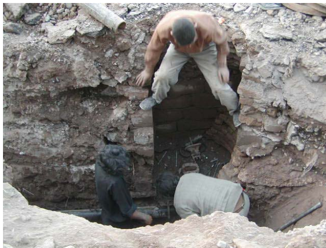
Photo 2.2.1 Damaged Qanat
