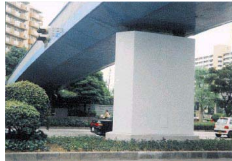
Figure 6.3.8 Example of Steel Jacketing Method
