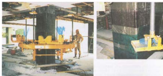
Figure 6.3.9 Example of Fiber Jacketing Method
