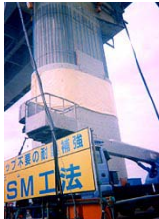
Figure 6.3.7 Example of RC Jacketing Method
