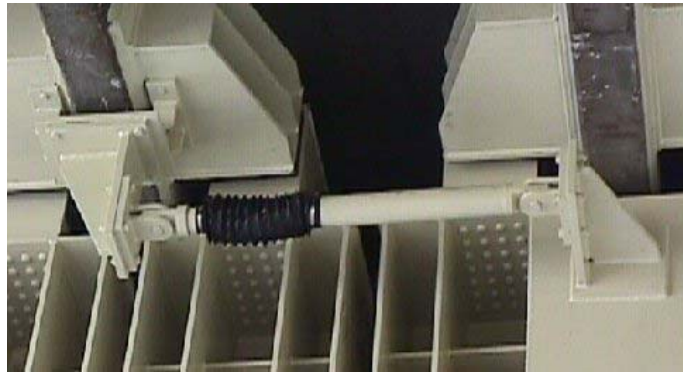
Figure 6.3.4 An Example of Displacement Controlling by Damper
