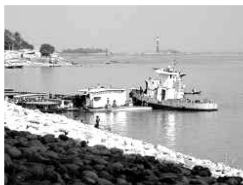
River Training Works of Bhairab Bridge
