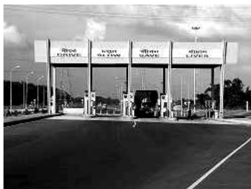
Toll Gate of the Paksey Bridge
