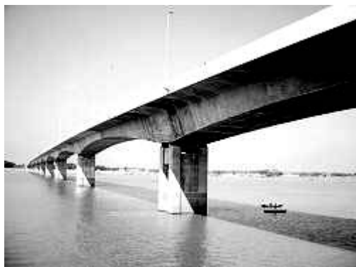
Main Bridge of Bhairab
