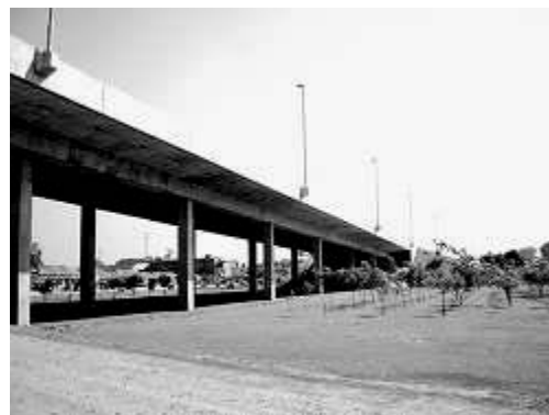
Viaduct of Bhairab Bridge
