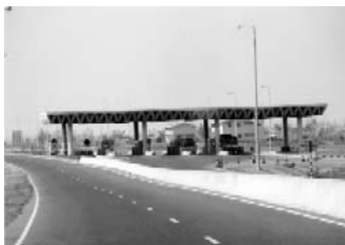
Toll Gate of Jamuna Bridge
