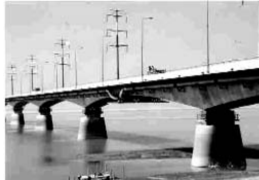
Encroachment (Gas Pipe Line)
