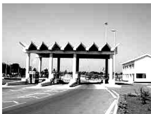
Toll Plaza of Bhairab Bridge
