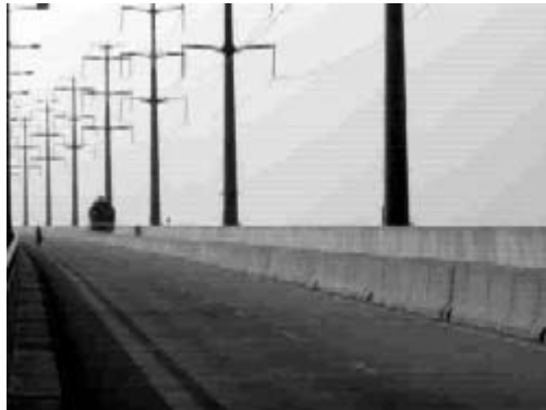
Encroachment (Electricity Posts)
