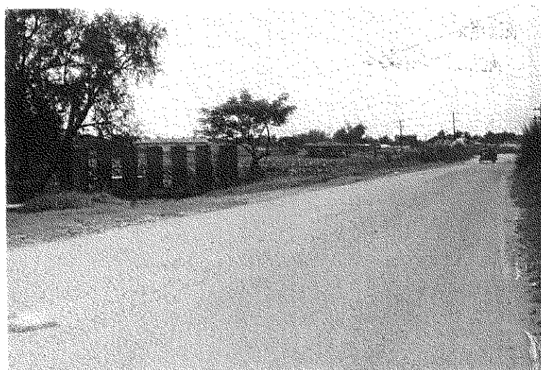
Brgy. Sto. Rosario, Sto. Tomas Pao Flood-Prone Area
