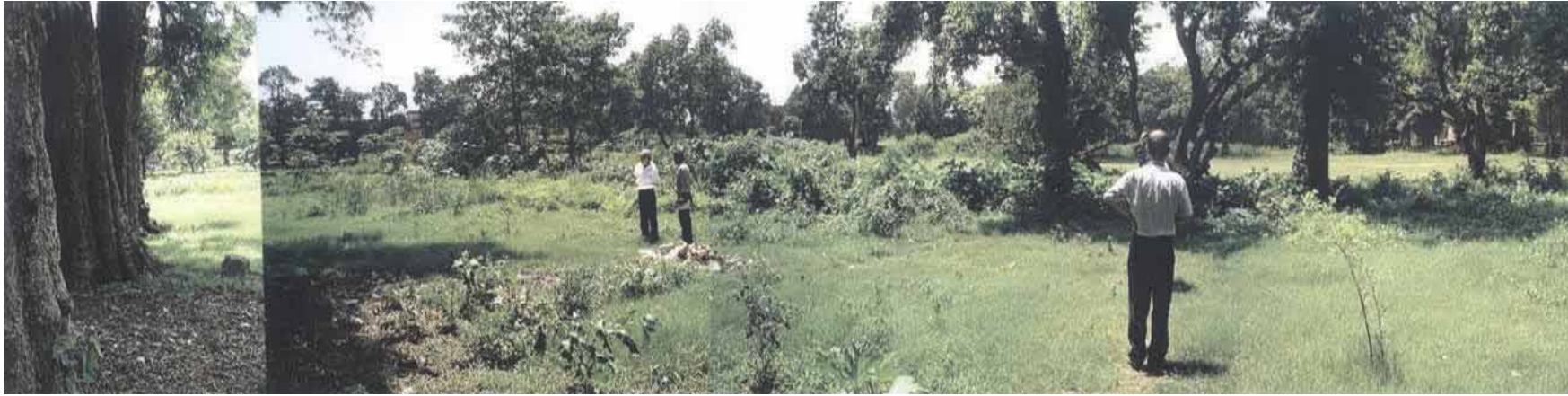
CONSTRUCTION SITE (Toward TANK from OPD WARD)
