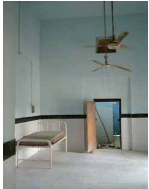
OLD MEDICAL WARD (UNDER REPAIRS)
