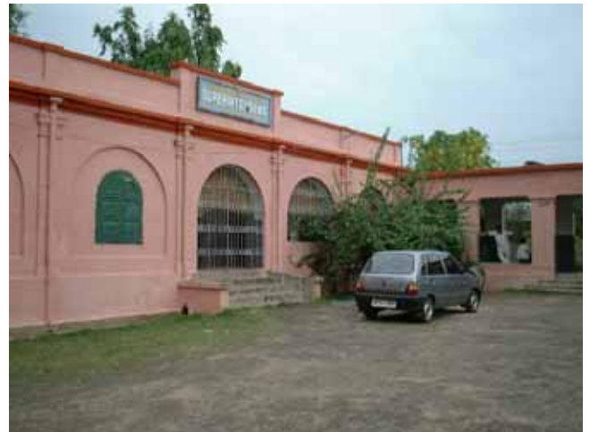
SUPERINTENDENT'S OFFICE (NORTH SIDE)
