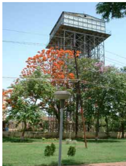
WATER TANK TOWER
