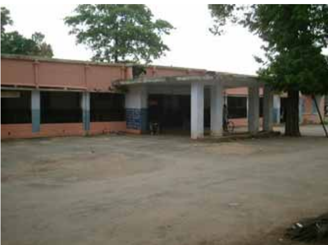
OPD WARD (SOUTH SIDE: MAIN ENTRANCE)
