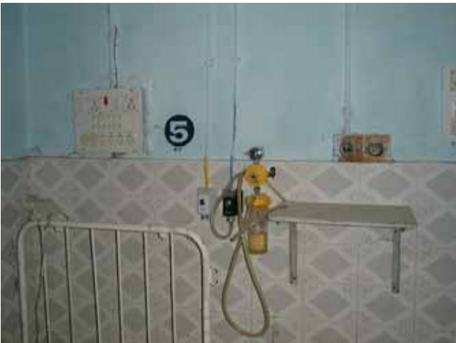
OLD MEDICAL WARD (ICU UNDER REPAIRS)
