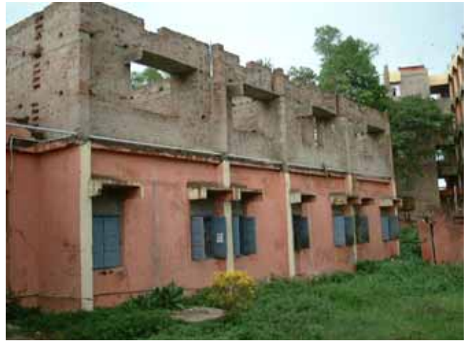
NEW MEDICAL WARD (EAST VIEW) (1ST FLOOR CONSTRUCTION SUSPENDED)
