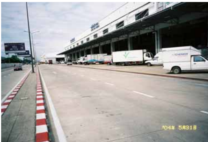
No. 18 Truck Docks of the Bonded Warehouse of Bangkok International Airport (2)
