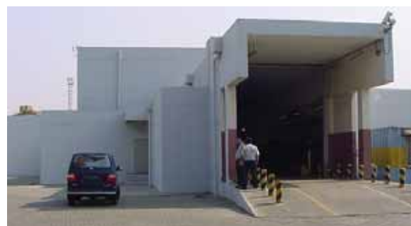
Entrance Gate of X ray Test Facility at JICT
