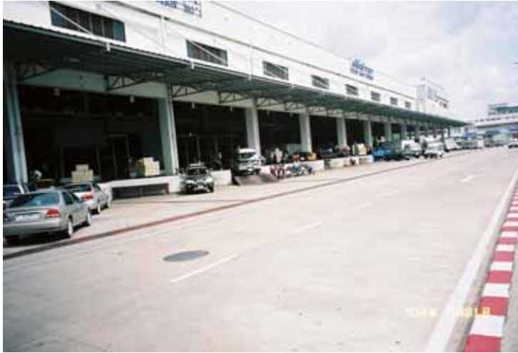
No. 17 Truck Docks of the Bonded Warehouse of Bangkok International Airport (1)
