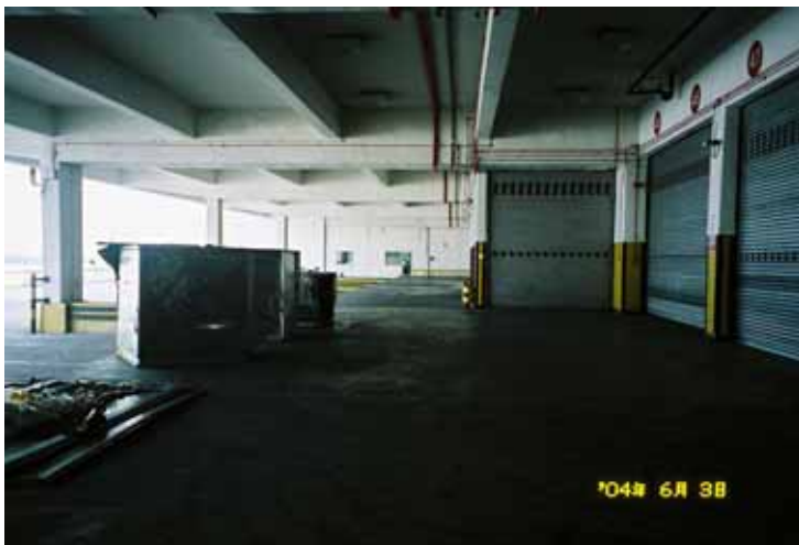
No. 21 Truck Docks of the Bonded Warehouse of Kuala Lumpur International Airport (2)
