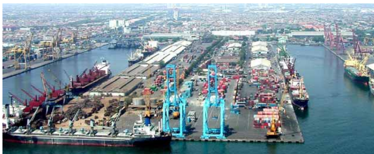
New Container Berth of Seguro at tip of Pier No 3, JICT 1 on left and JICT 2 on right side.
