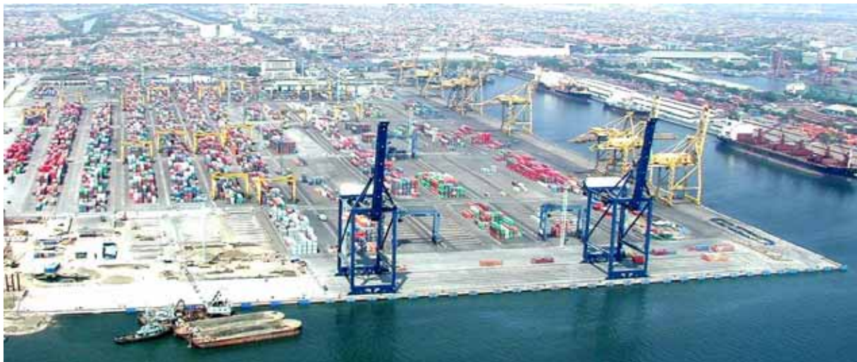
Jakarta International Container Terminal 1 (JICT 1) North berth and West Berth at 2003
