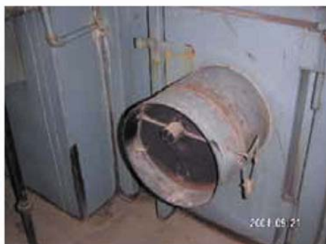
Draft vane & Dust removal
