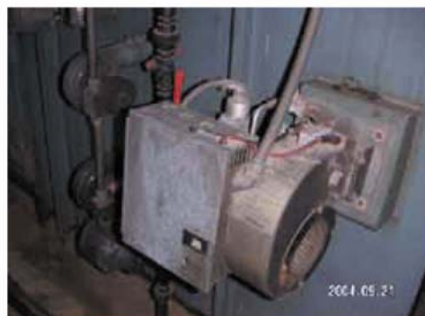
Auxiliary burner
