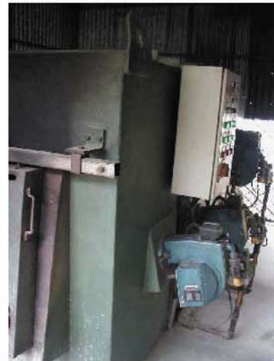
1st buffer wall
