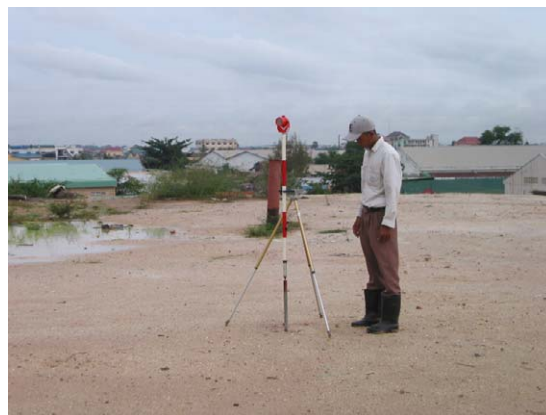
Photo: Measurement of settlement
