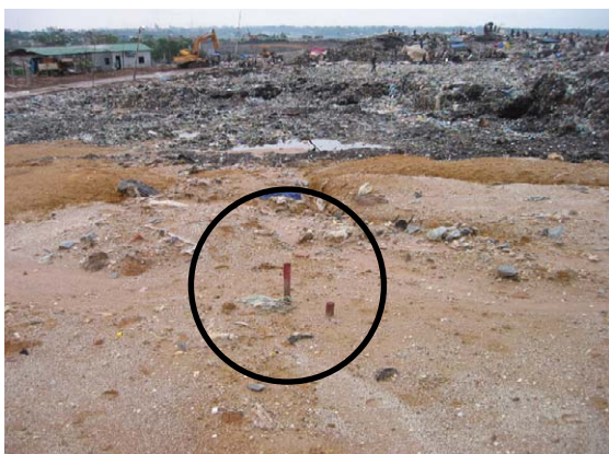
Photo: Settlement board
