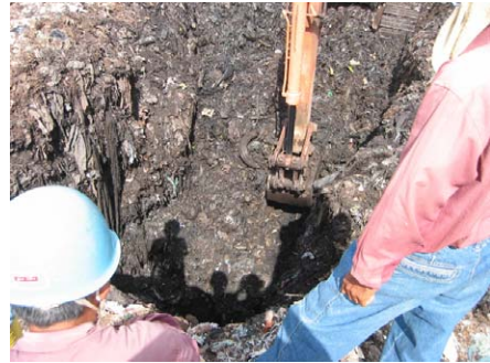
Photo: Excavation (backhoe)
