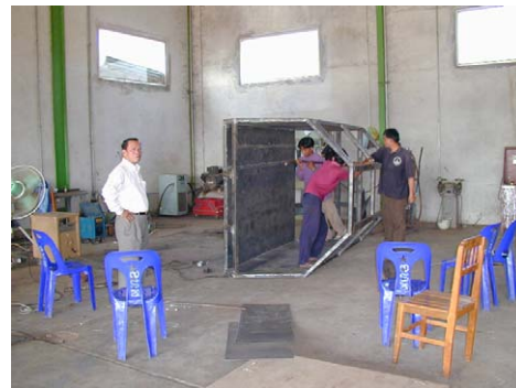
Construction of container at maintenance shop
