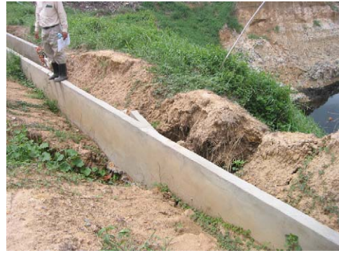
Broken Drain 3
