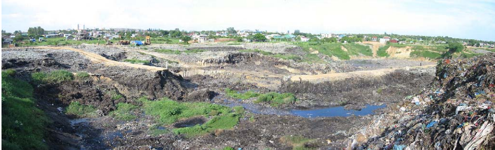
Scene of the Bank-C collapse from inside of the expansion area
