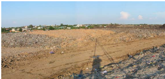
After final covering
