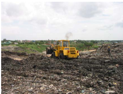
Spreading work of waste
