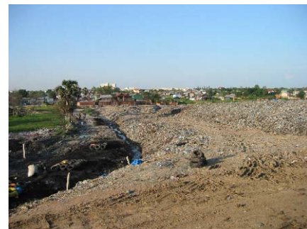
After spreading work
