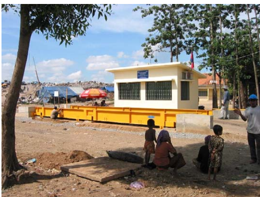
Construction of Weighbridge
