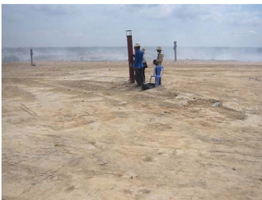
Model Block and Gas Removal Pipes
