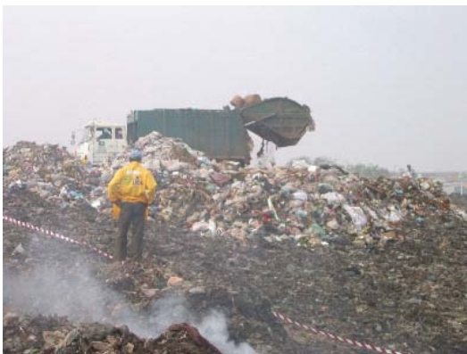
Working Area Separation (Waste Unloading Area)
