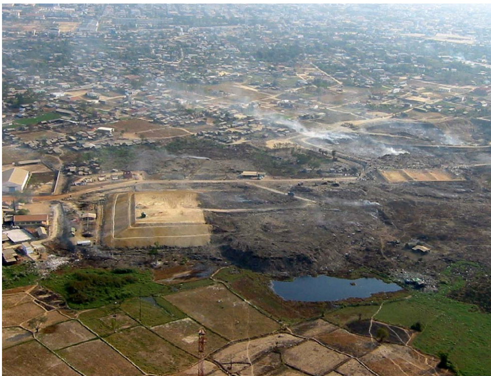
SMC Disposal Site after Pilot Project (March 2004)
