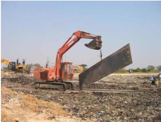
Construction of Working Face
