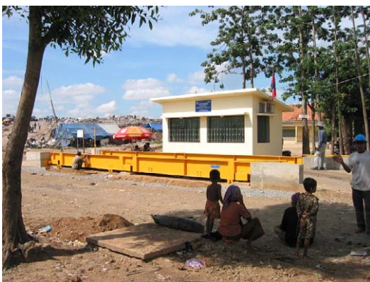
Construction of Weighbridge
