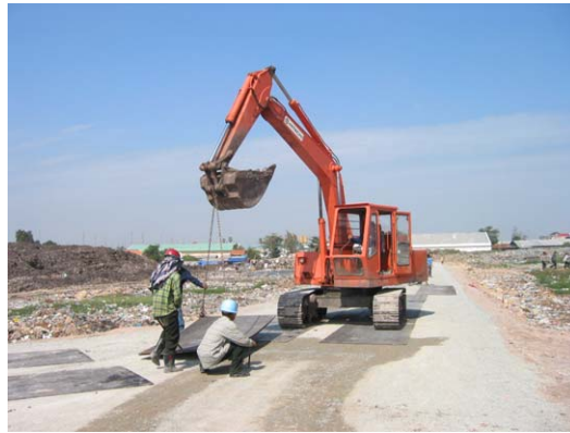
Construction of Main Road
