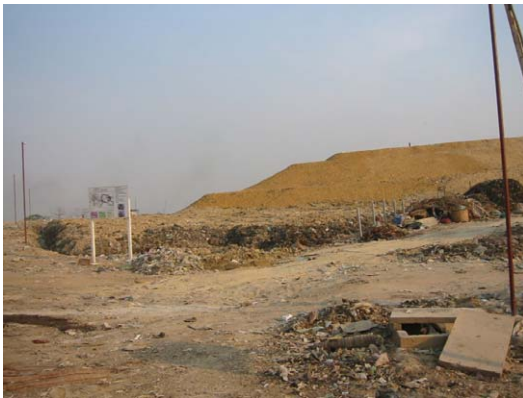
Construction of Model Block
