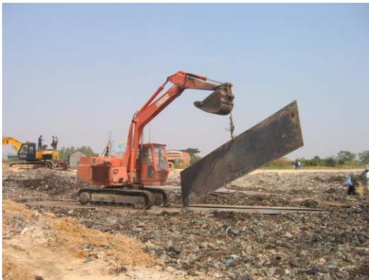
Construction of Working Face
