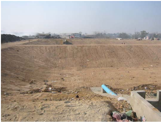
Leachate Treatment Pond (Under Construction)
