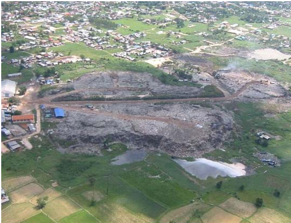
SMC Disposal Site before Pilot Project (September 2003)
