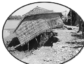
Bank erosion and damage to housings
