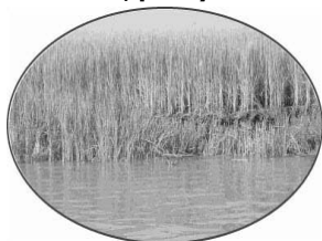
Bank erosion and damage to paddy field
