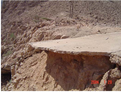
Road failure at Wadi
