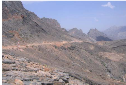
Landscape of N27 Project northeast of Jabal Shams
