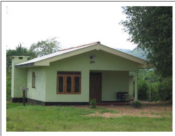
Completion in March 2004 [Galpaya Vidyalaya]
