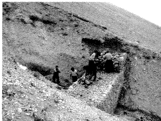
Construction of a gabion check dam
