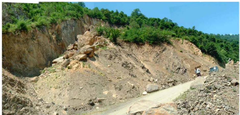
Photo A2.2.1.3 Landslide at Upstream of the Masulero River (Colluvial deposit type landslide)
