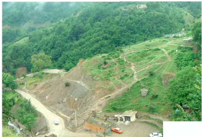
Photo A2.2.1.4 Landslide at Masuleh Town (Weathered rock type landslide)
