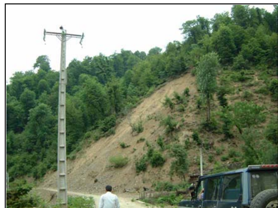
Photo A2.2.1.1 Slope Collapse at Upstream of the Chafroud River
