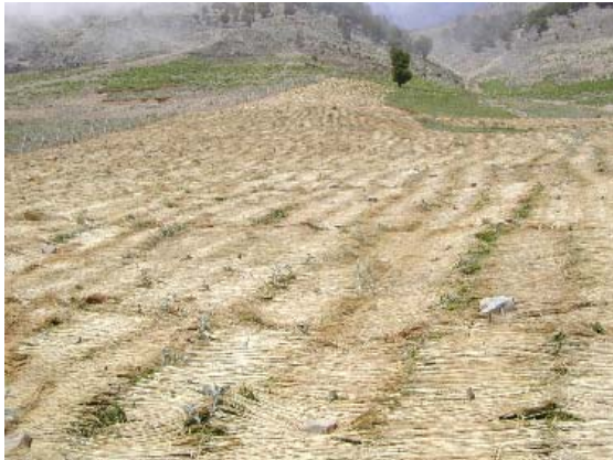
Straw matting to control erosion in Upper Masuleh
