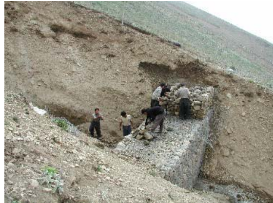
Construction of a gabion check dam
