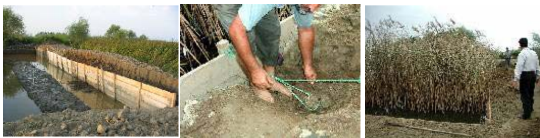
Figure 12.3.22 Reed Bed during Construction
