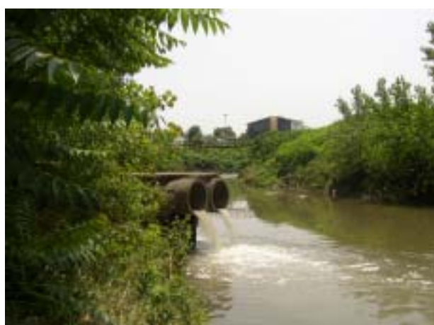
Discharge of Wastewater without Treatment
