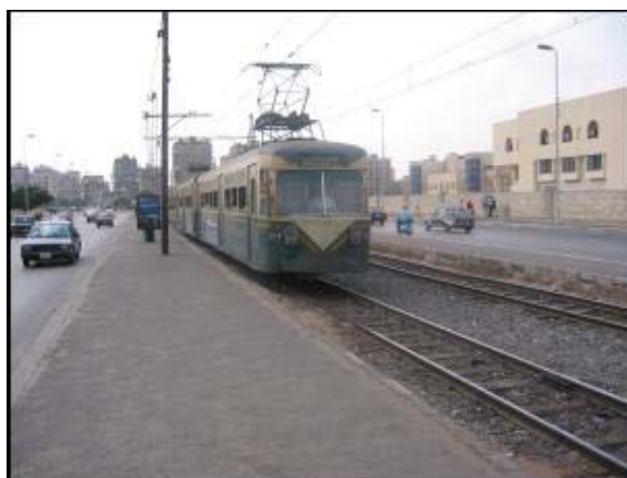
Figure 3.1.3 Typical central Right-of-way between Abdel Al-Magid Salim Bridge and Madinet Nasr Terminal
