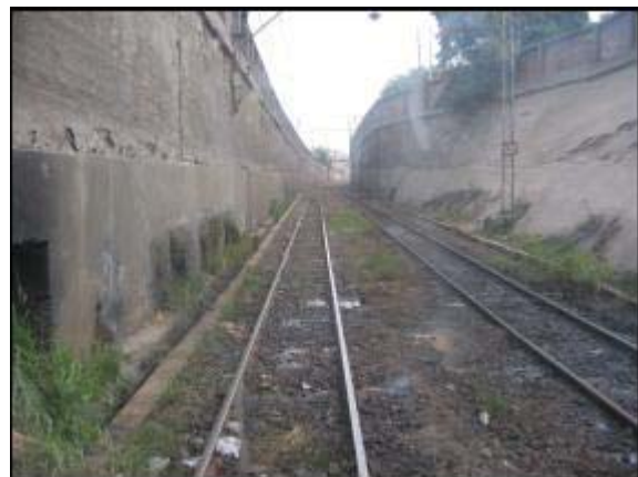
Retained cut lateral right-of-way
