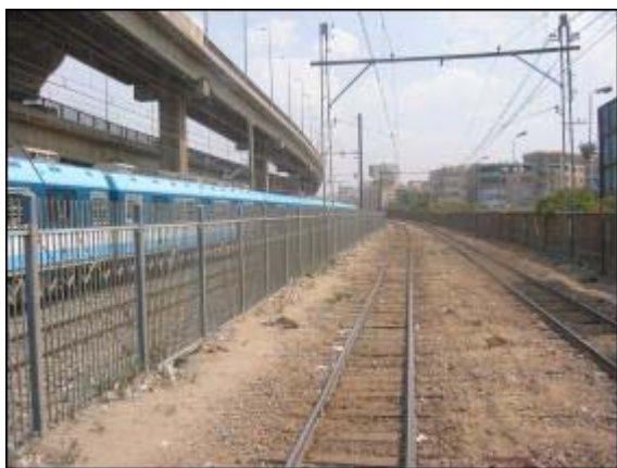
At grade lateral right-of-way
