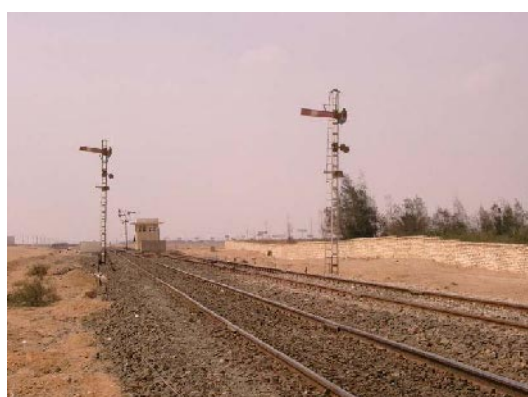
Photo - 2 Signal System
