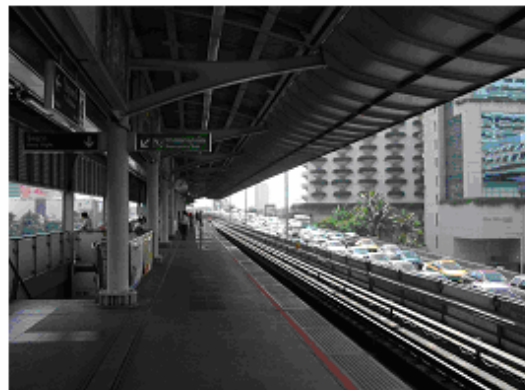
Photo-2 Elevated Platform
