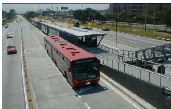
Figure ES.10 A Busway System in Colombia
