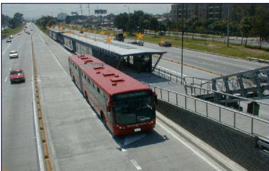
Figure A-2-1 A Busway System in Colombia
