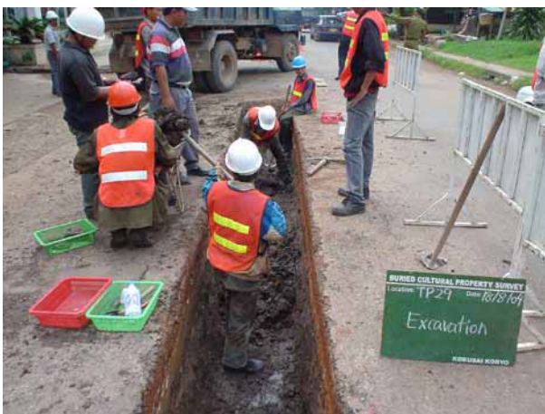
Excavation in progress
