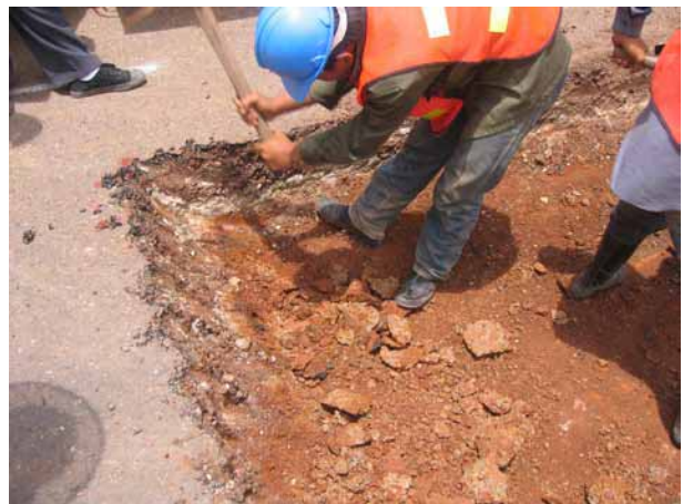
Excavation in progress
