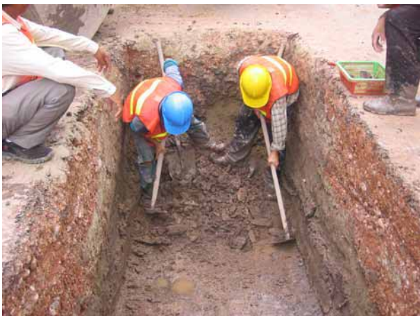
Excavation in progress
