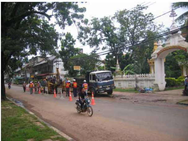
Site of the excavation
