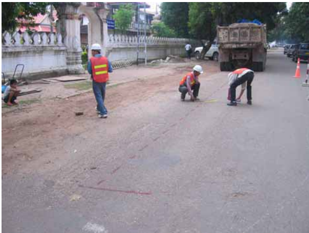
View of the excavation site
