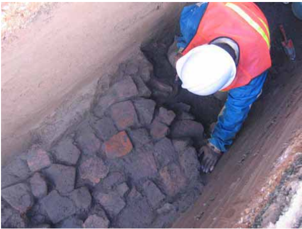
Excavation under progress
