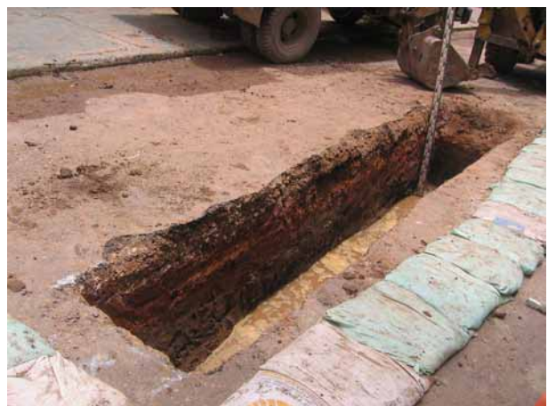
Colonial-era brick foundation
