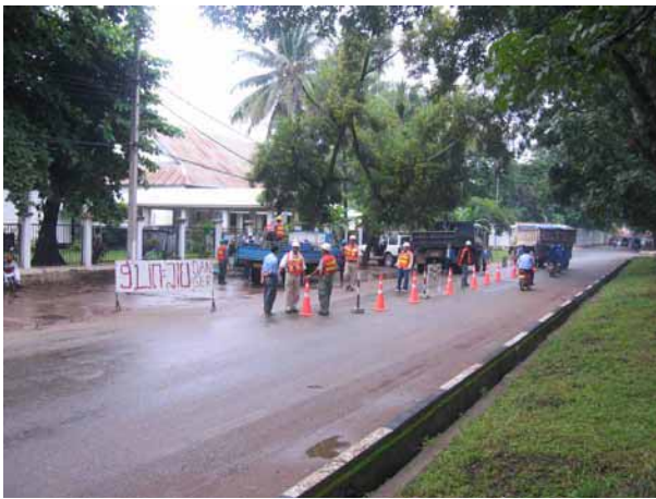
Site of the excavation
