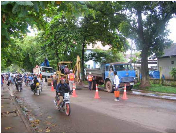
View of the excavated area
