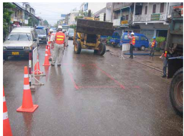
Excavation in progress
