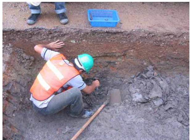
Excavation in progress
