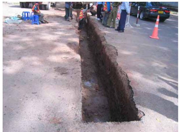
Test Pit 27 after excavation
