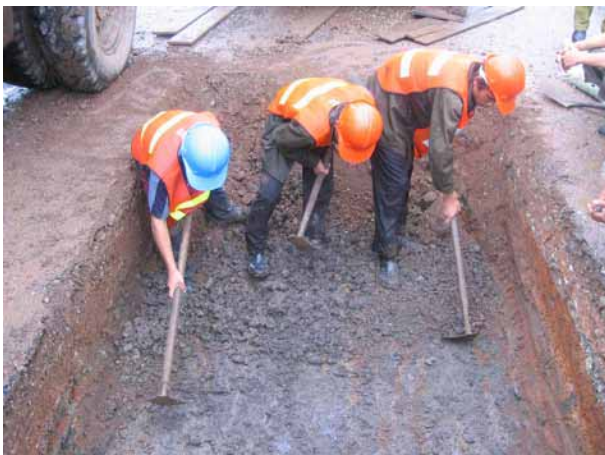
View of the excavated area
