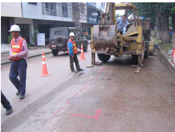
Site of the Test Pit 32
