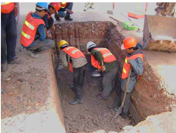
Excavation in progress
