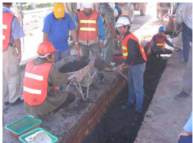
Colonial-era brick foundation
