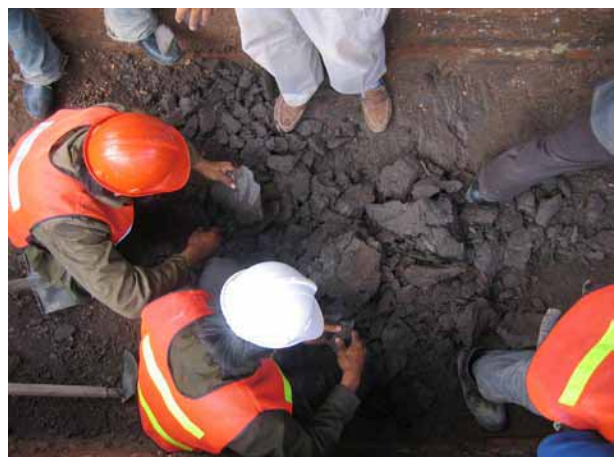
Excavation in progress
