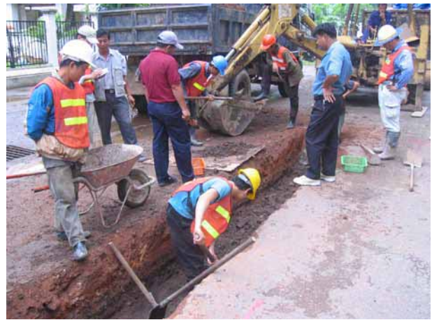
Excavation in progress
