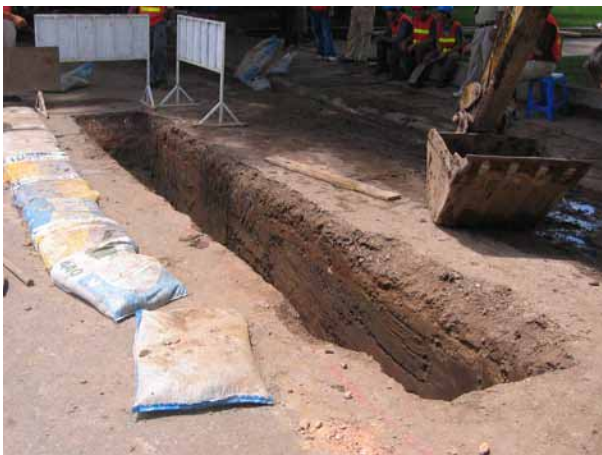
View of the Test Pit after excavation
