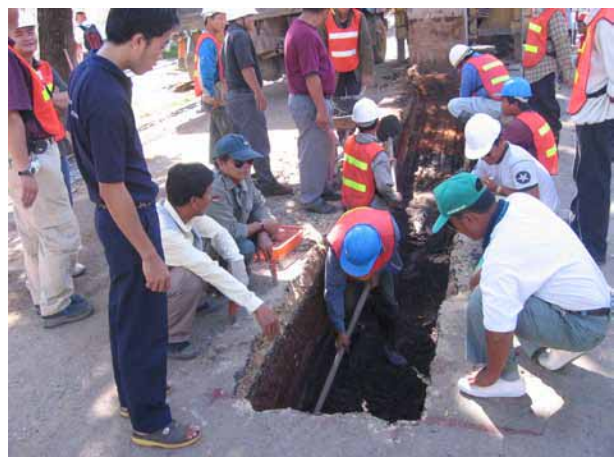
Colonial-era brick foundation
