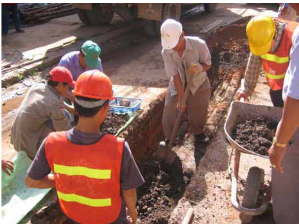
View of the test pit after excavation
