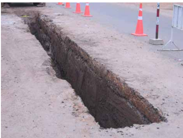
View of the test pit after excavation
