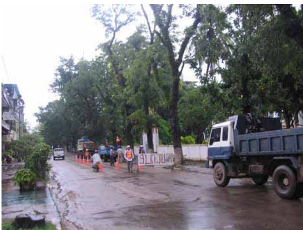
Site of the excavation
