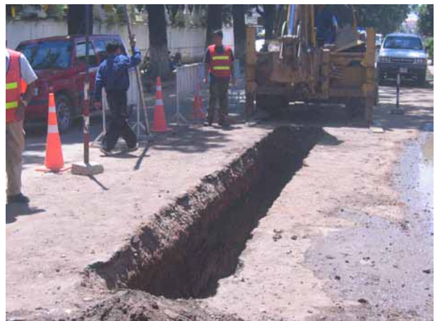
Colonial-era brick foundation
