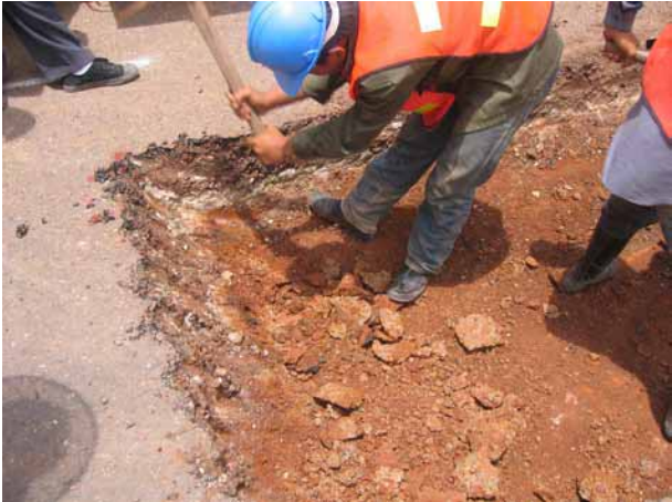
Excavation in progress
