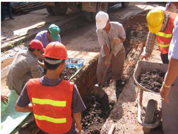
View of the test pit after excavation
