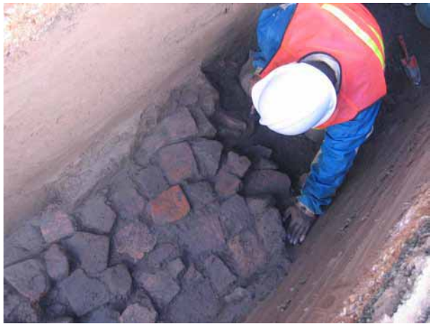
Excavation under progress
