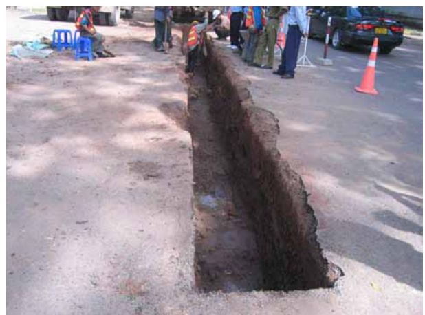
Test Pit 27 after excavation
