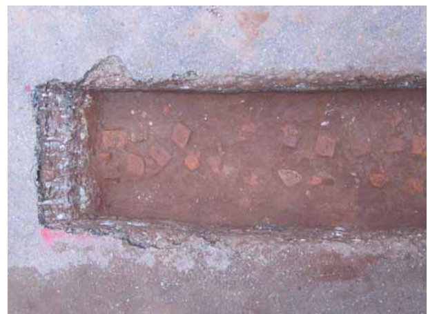
Alignment of bricks
