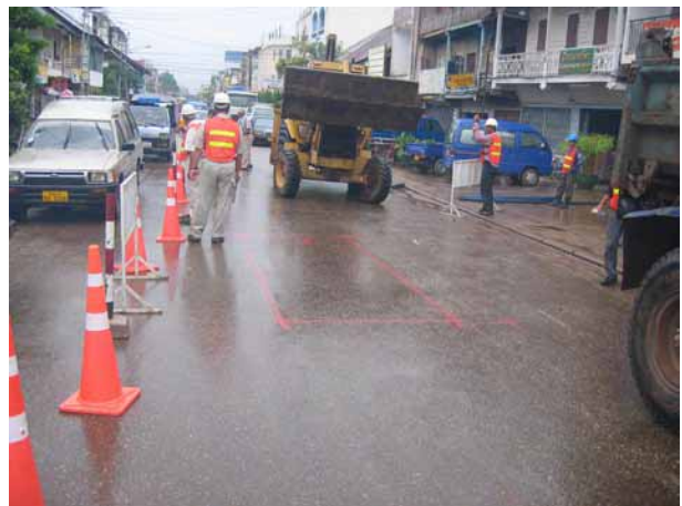
Excavation in progress
