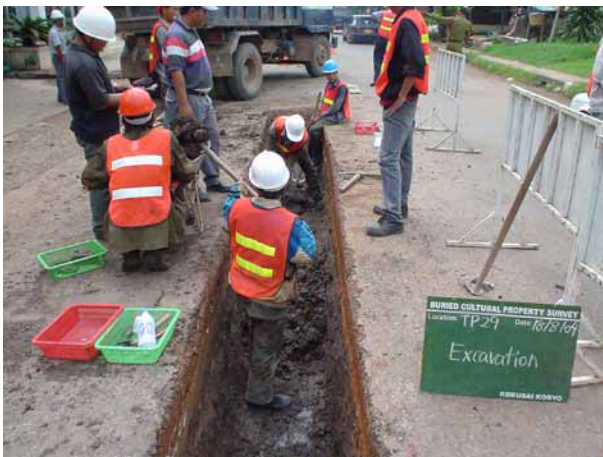
Excavation in progress
