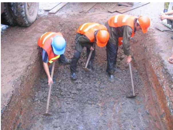
View of the excavated area
