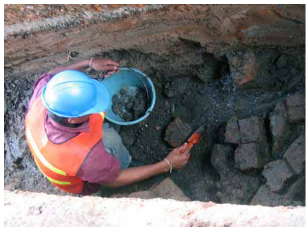
Excavation in progress
