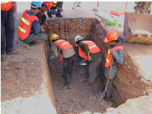
Excavation in progress
