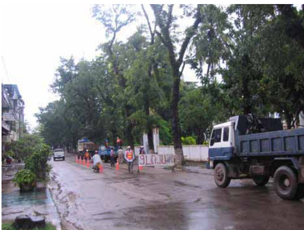
Site of the excavation
