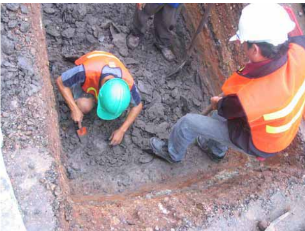
Excavation in progress
