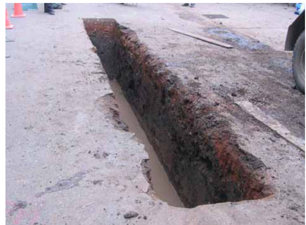
View of the Test Pit 28 after excavation
