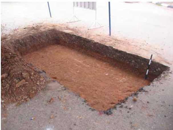
Old brick pavement
