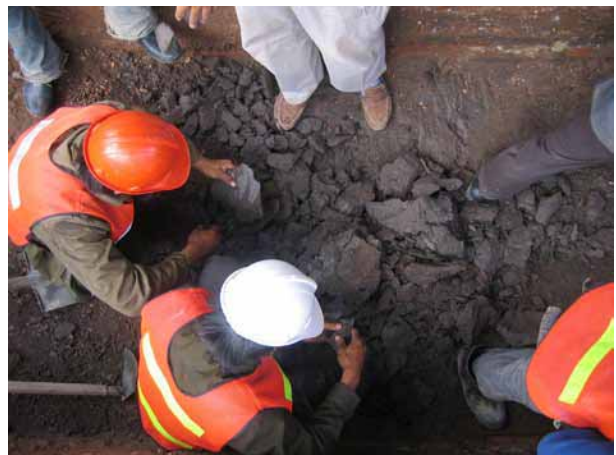
Excavation in progress
