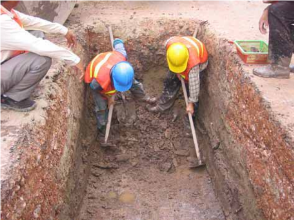
Excavation in progress
