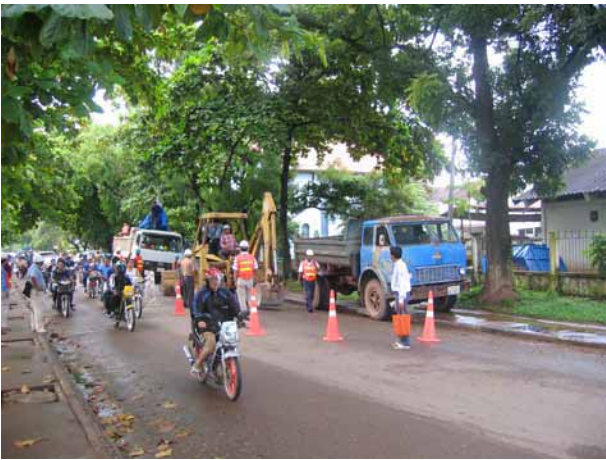
View of the excavated area
