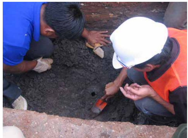
Excavation in progress
