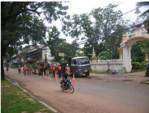
Site of the excavation
