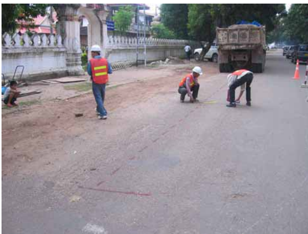
View of the excavation site
