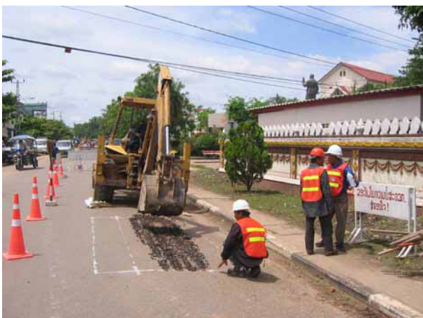
Removing asphalt at Test Pit 08
