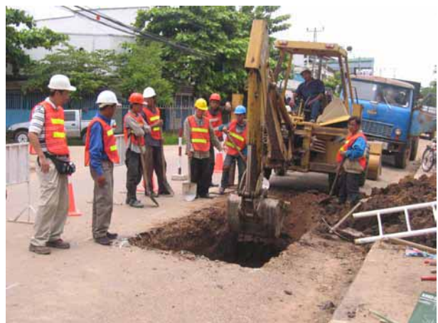
Deeper excavation by mechanical shovel
