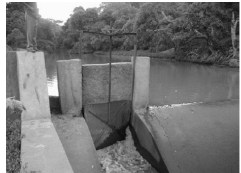
Scouring sluice gate
