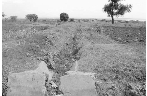
Secondary canal (Gidano II)
