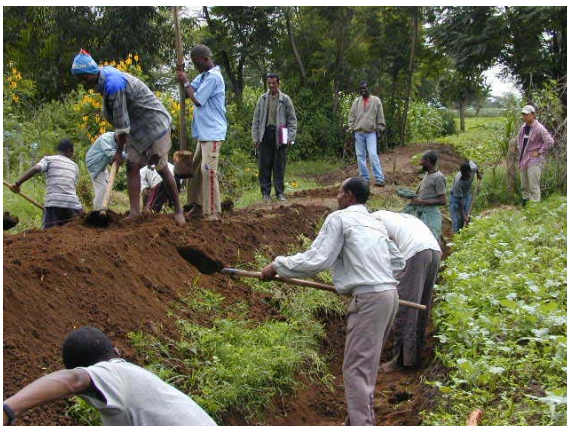
Participatory Work of Irrigation Canal (Oda Chisa WUA)
