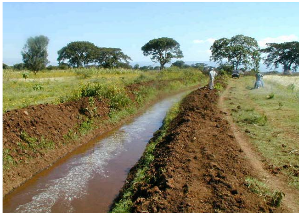
Main Canal after Clearing of Sedimentation
