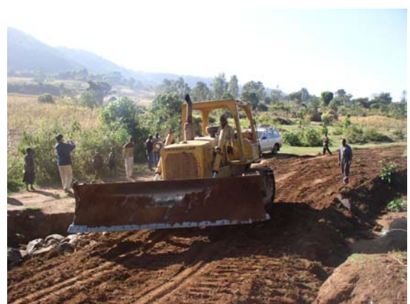
Rehabilitation Work by Heavy Equipment of OIDA
