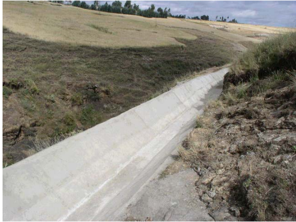
Main Canal after Plastering Works (Water Loss was largely improved, Nov 2003)
