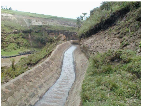
Main Canal before Rehabilitation Works (Oct 2003)
