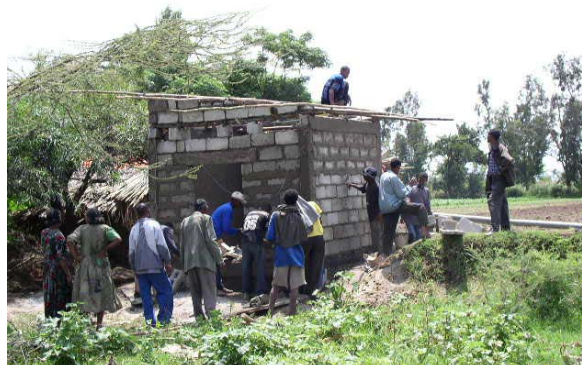
Participatory Work of Pump House
