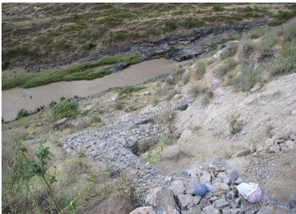
Provision of Gabions for Slope Protection
