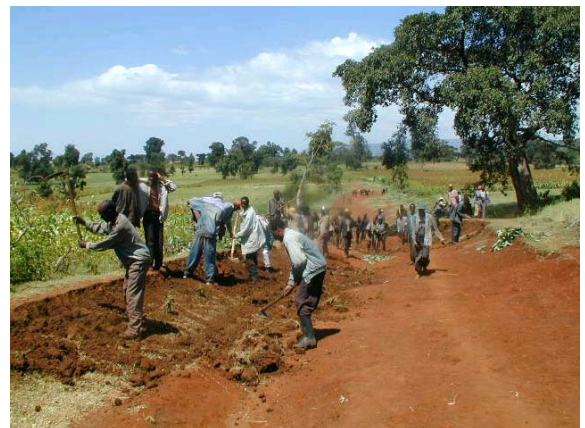
Repair of Gully by Community People
