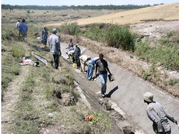
Plastering Works in Cooperation with WUA Members
