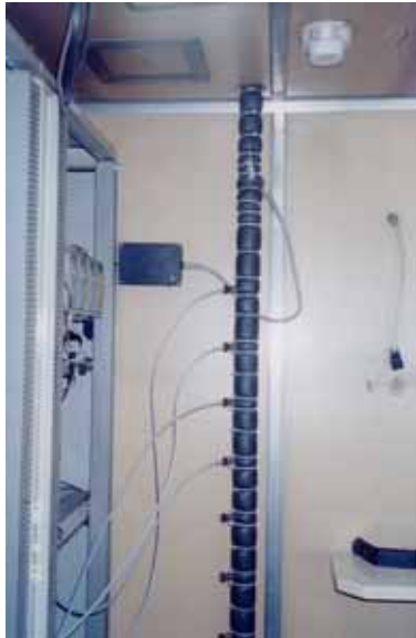
Figure 6 Vertical Manifold with thermal insulation
