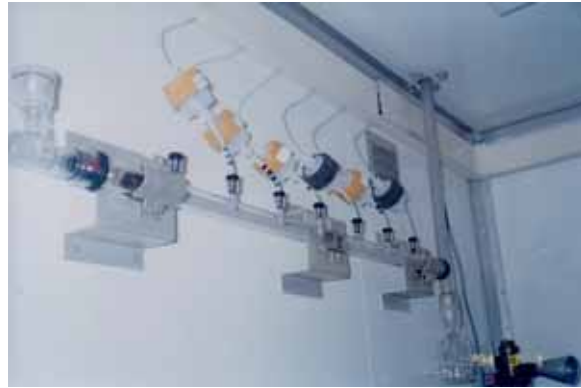
Figure 7 Horizontal Manifold with thermal insulation
