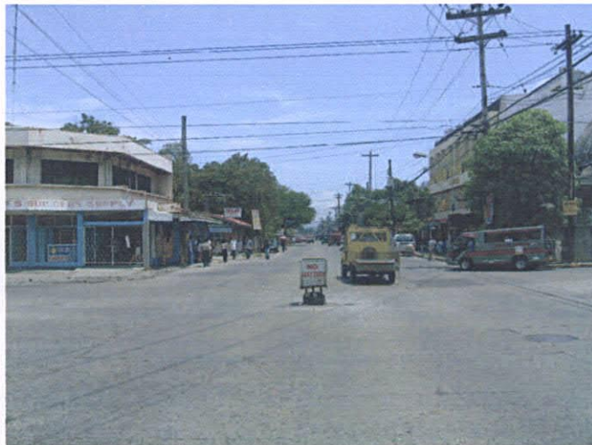
FIGURE 4.3-8 "NO LEFT TURN" SIGNBOARD AT INTERSECTION
