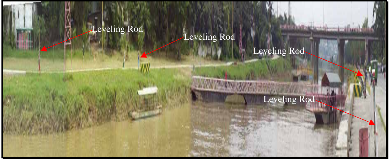
Location of leveling rod, which will serve as starting and end point of the float
