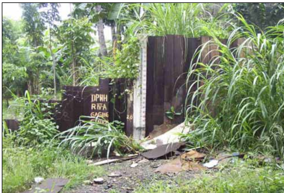
Existing Gauging Station at San Cristobal River
