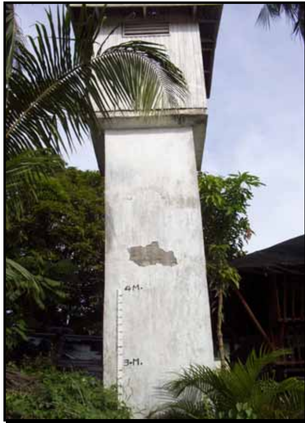
Existing Gauging Station at Brgy. Poblacion along Pansipit River
