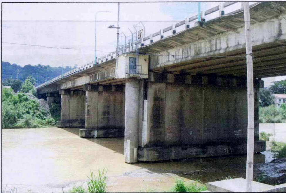
Existing Gauging Station at Montalban Bridge, Montalban Rizal
