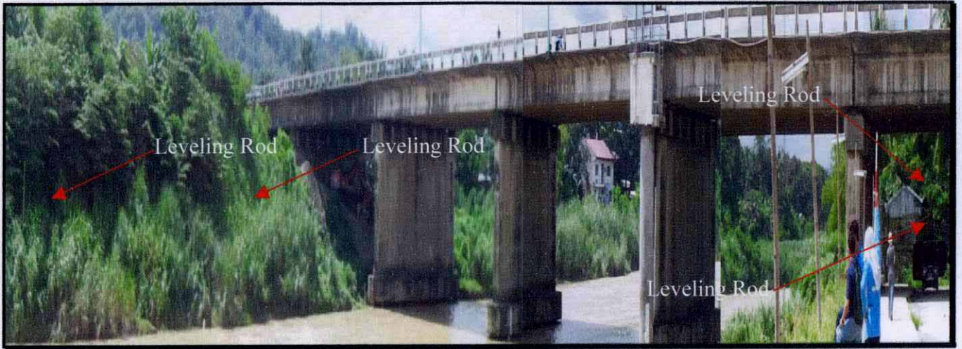
Location of leveling rod, which will serve as starting and end point of the float
