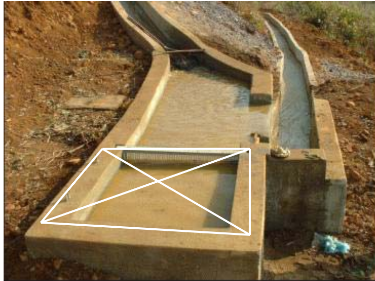
Figure 3-13 A head tank and a spillway (right side)
