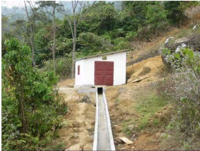
Figure 3-26 A powerhouse and tailrace
