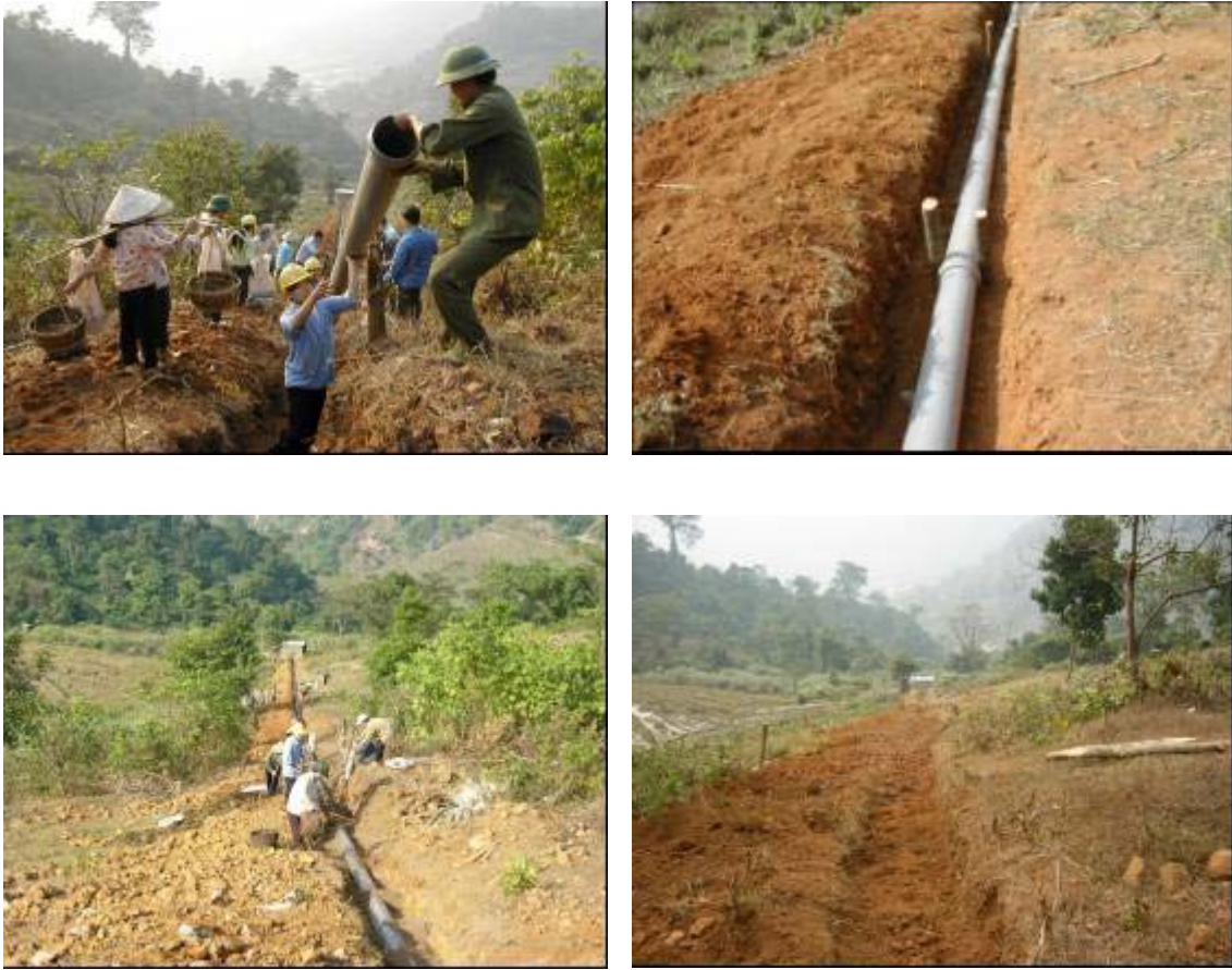
Figure 3-21 Installation of a PVC penstock
