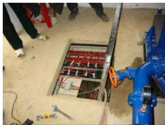
Setting dummy load in tailrace
