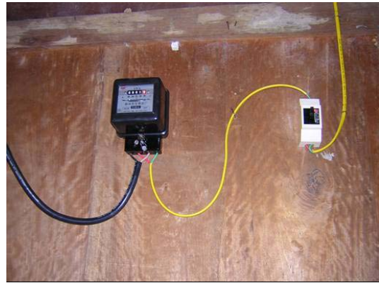
Figure 3-5-2 House connection (Left:Lead-in wire and post, Right:Watt-hour meter and circuit breaker)
