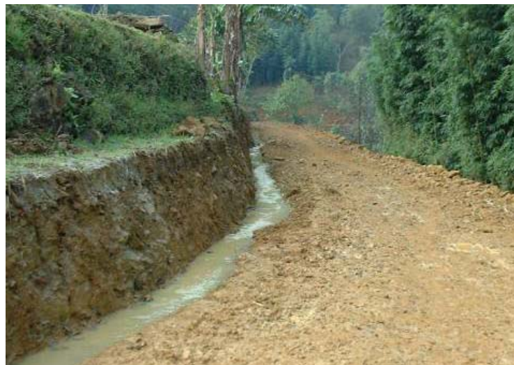
Figure 3-3-3 The existing channel after renovation
