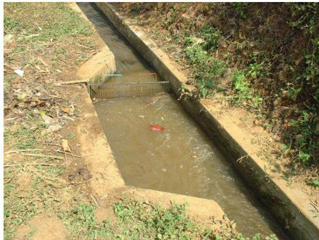
Figure 3-3-6 The silt basin
