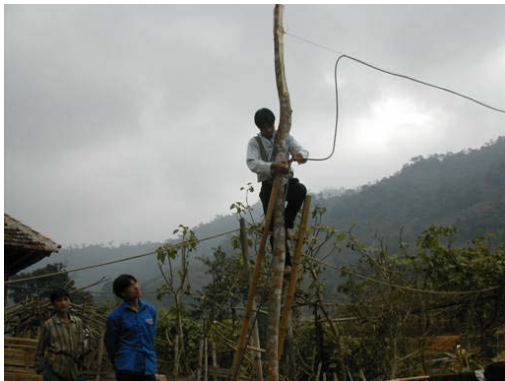
Figure 3-5-3 Installation of lead-in wire
