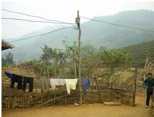
Figure 3-5-2 House connection (Left:Lead-in wire and post, Right:Watt-hour meter and circuit breaker)
