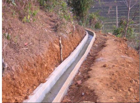
Headrace (newly built)
