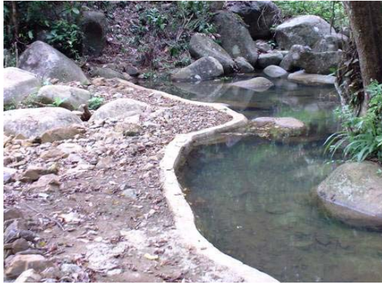
Figure 3-3-1 The weir and intake after renovation
