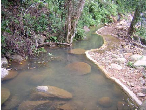
Intake weir (renovated by villagers)
