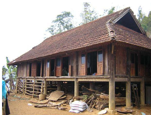
Figure 1-4 A typical house in Theu
